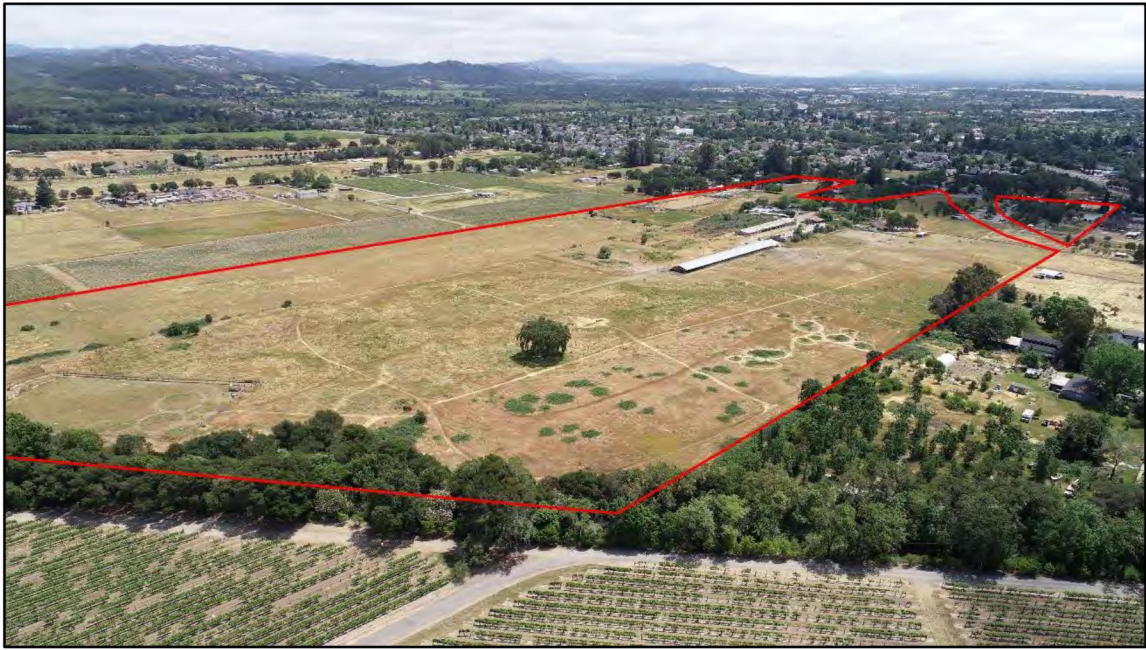
5a-1: Looking southeast from northwest corner. Photo Date 5-24-18
