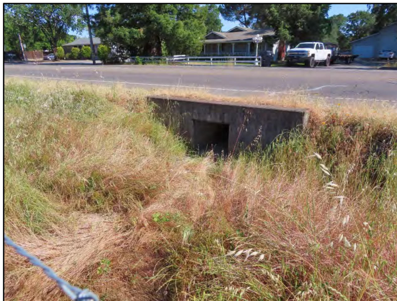
Box culvert under Arata Lane. Water drains from roadside ditch through this culvert. Photo date 5-6-21
