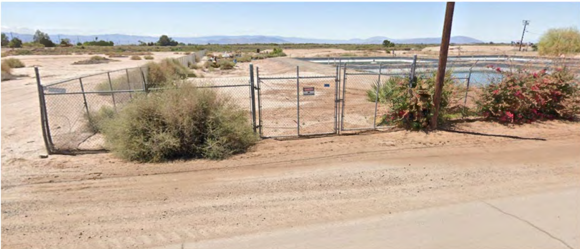
Figure 3-2 View of the SCWD WWTP from New River Boulevard
