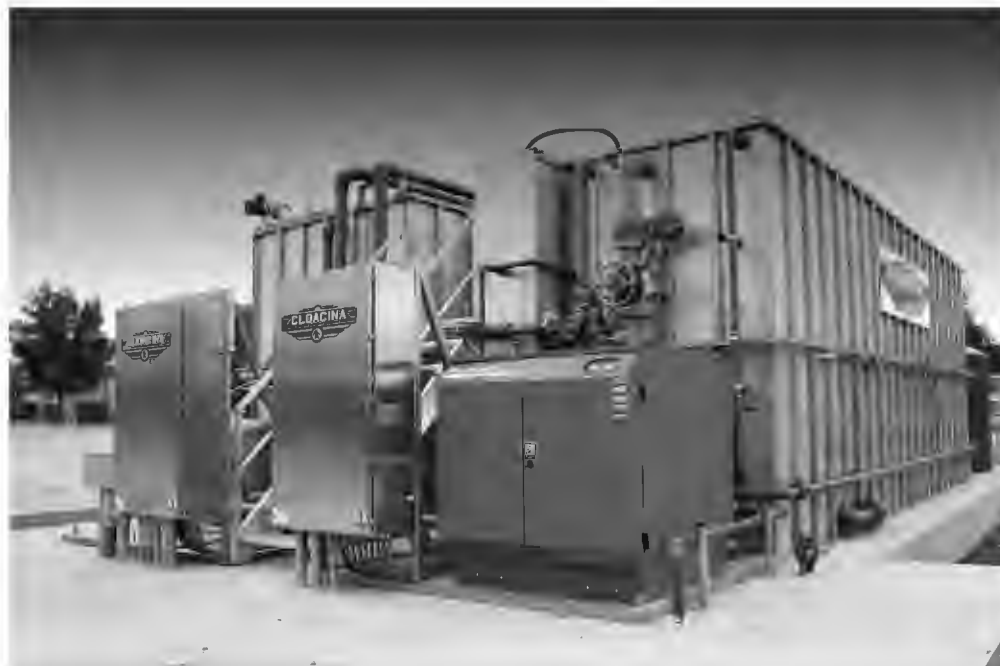
Figure 4-2: Typical Package MBR Installation (Courtesy Cloacina)
