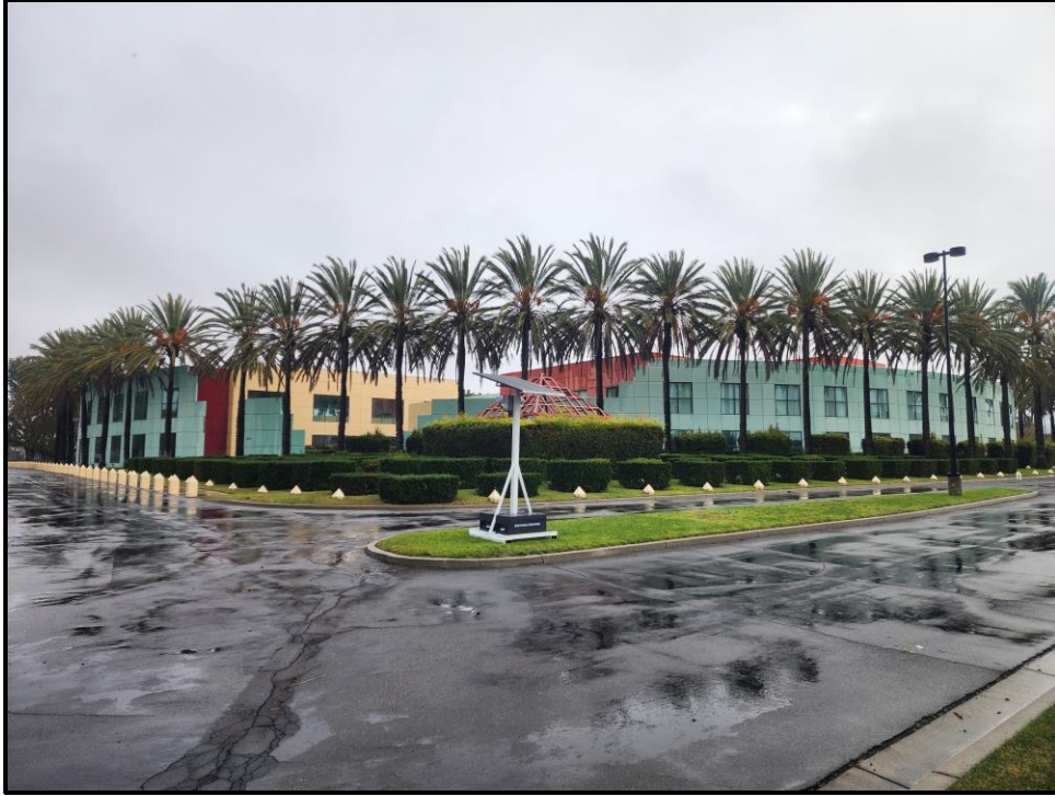
Plate 3.2-1: An overview of the project, facing northeast.
