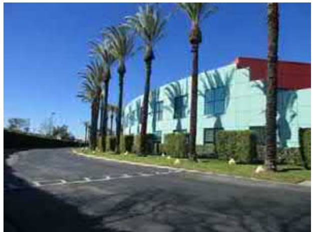
10. View of the southwestern portion of the subject property facing north.
