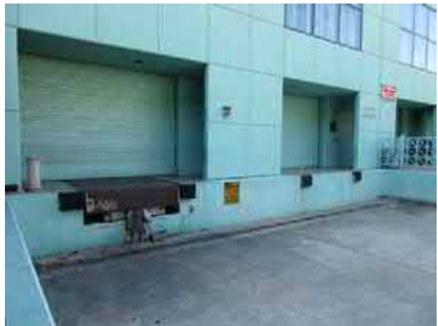
58. View of dock and sump pump located on the eastern portion of the subject property.
