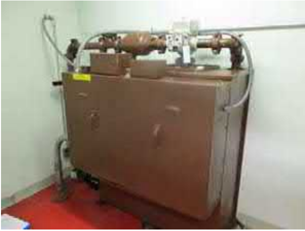
31. View of elevator equipment found on the subject property.
