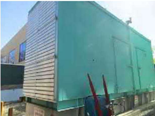
53. View of diesel containment area on the eastern portion of the subject property.
