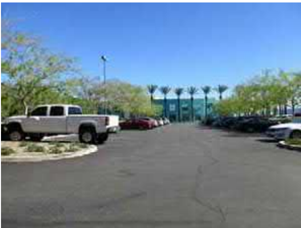
15. View of the northern portion of the subject property and general parking facing south.
