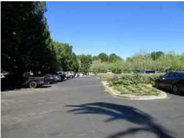
17. View of the asphalt paved parking area of the subject property facing east.
