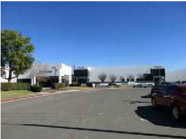
65. View of adjacent property to the south facing east.
