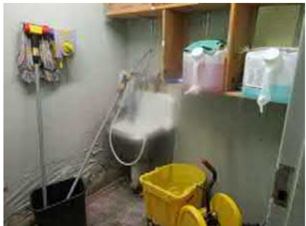
30. View of typical janitorial closet located on the subject property.
