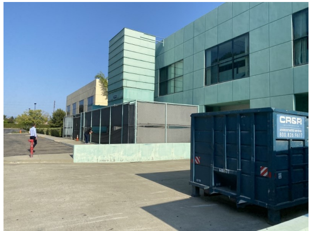
4.View of the subject property: loading dock
