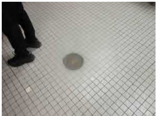
28. View of typical drain in kitchen in the subject property.
