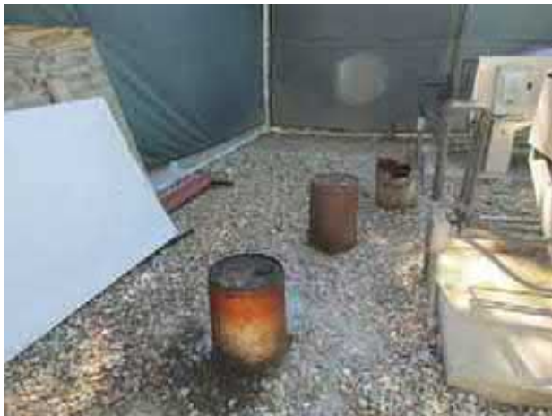
57. View of leaking oil barrel found near the systems cooling tower on the subject property.
