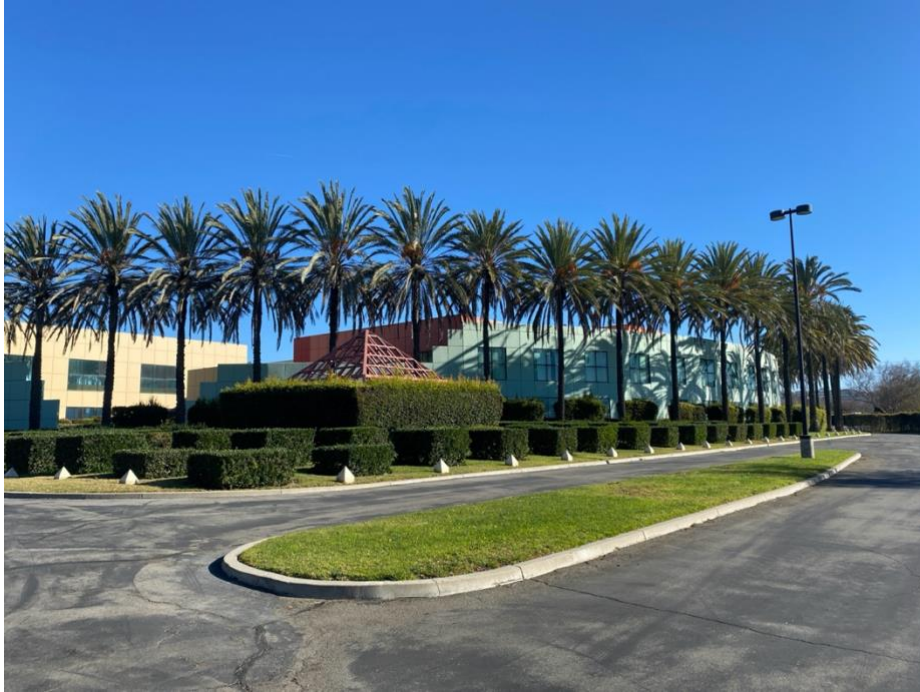
Photograph 5: Northeast-facing view of the existing buildings surrounded by landscaped ornamentals.
