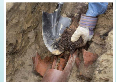
Plumber making repairs on private lateral
