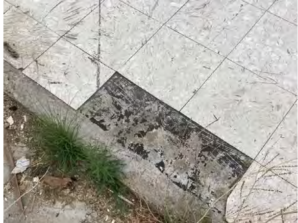
8 : Close up view of floor tile and black mastic on remnant foundation
