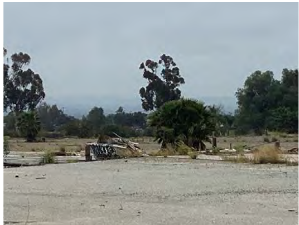
10 : View of Subject Property looking east
