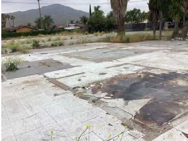
7 : View of floor tile and black mastic on remnant foundation
