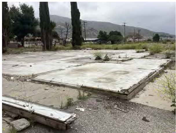
6 : View of the remnant foundation of a building
