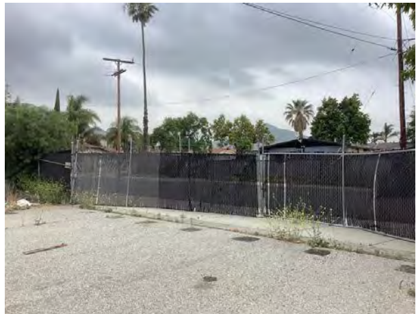
4 : View of the access gate along 33rd Street
