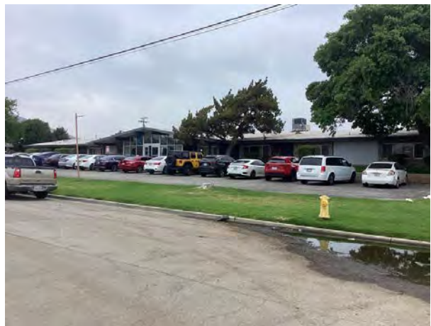
18 : View of northeast adjacent property (6401 33rd Street)
