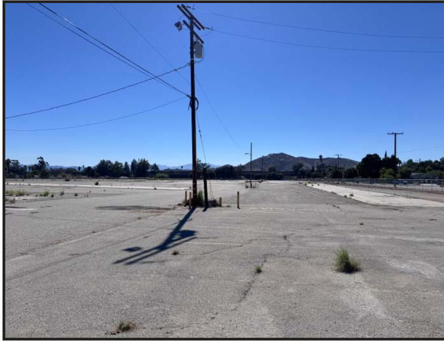
PHOTOGRAPH 1 - Southwest view of Project Site.
