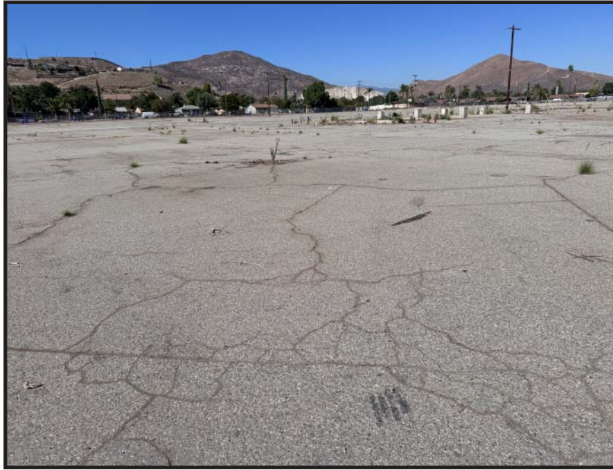
PHOTOGRAPH 3 - Northwest view of Project Site.
