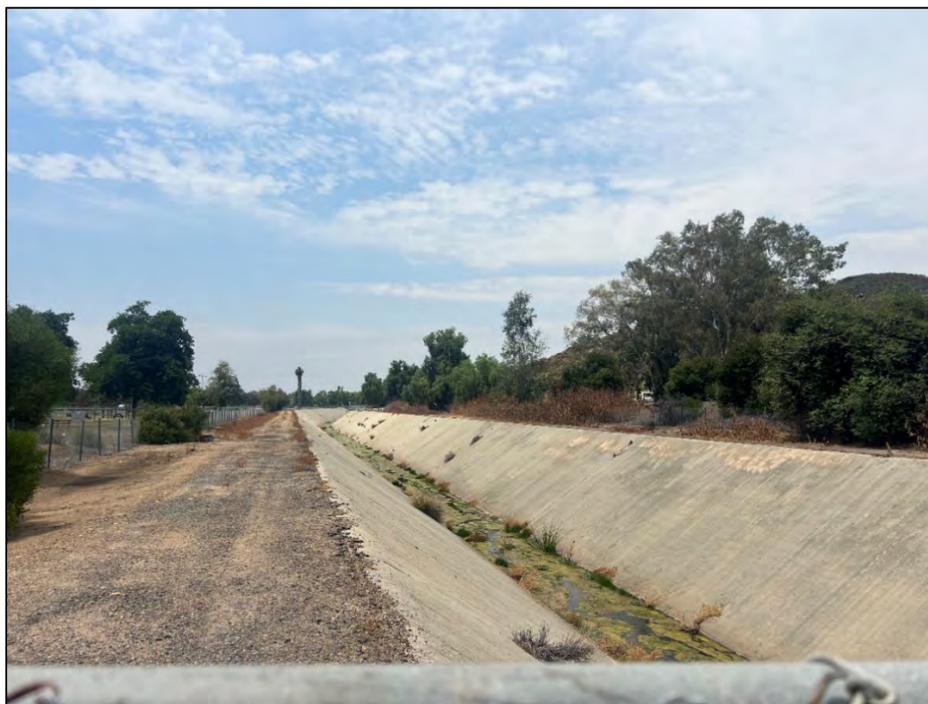
Photograph 2. View north of Escondido Creek from Beven Road.
