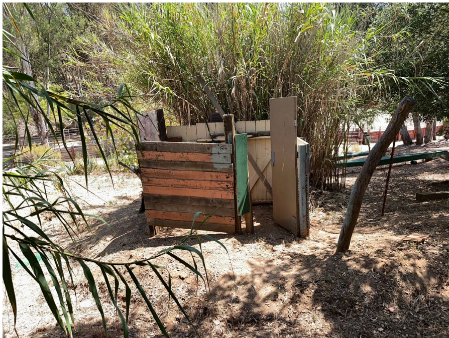
PHOTOGRAPH 8: SMALL MAKESHIFT CHANGING ROOM, BUILT IN 2016. VIEW NORTHEAST, JULY 17, 2024
