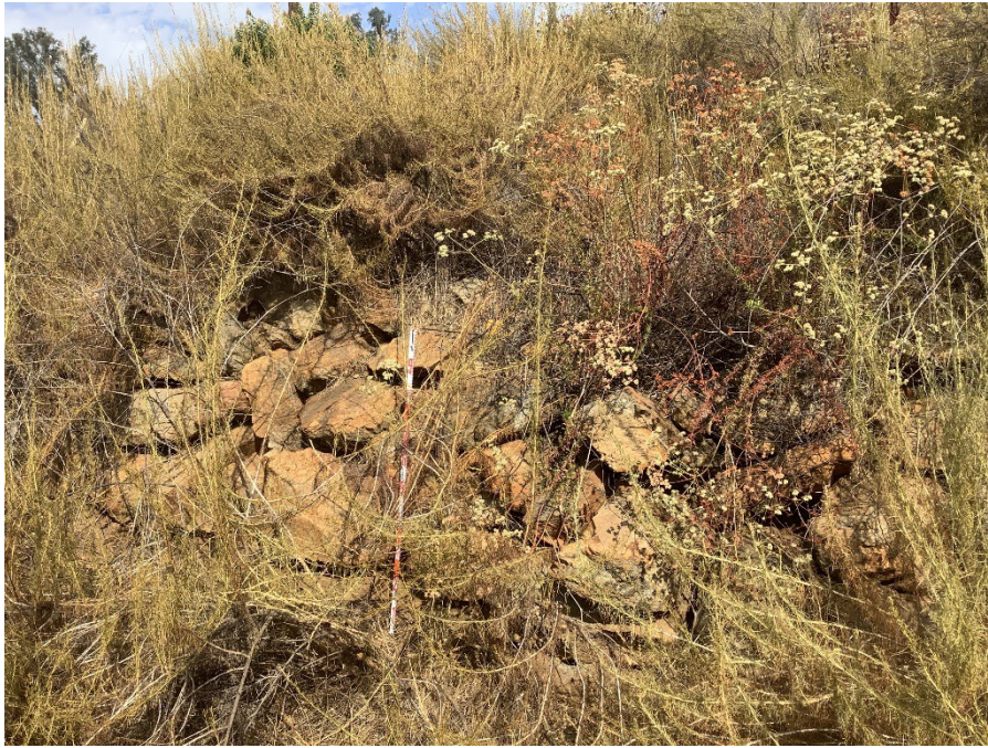
PHOTOGRAPH 12: ROCK RETAINING WALL FEATURE 3, ONE OF FOUR FEATURES IDENTIFIED DURING THE SURVEY.
