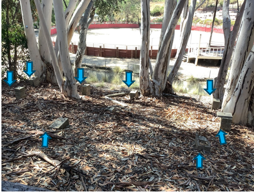
PHOTOGRAPH 3: OVERVIEW OF FOOTINGS FOR BENCHES INSTALLED IN 1974 FOR KEYHOLE ARENA. RED ARROWS POINT TO INDIVIDUAL FOOTINGS. VIEW SOUTHEAST, JULY 17, 2024.
