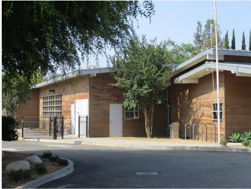
Photograph 14. East elevation of 3160 East Del Mar Boulevard, looking southwest.
