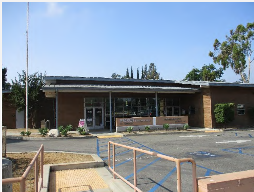
Photograph 13. Primary (north) elevation of 3160 East Del Mar Boulevard, looking south.
