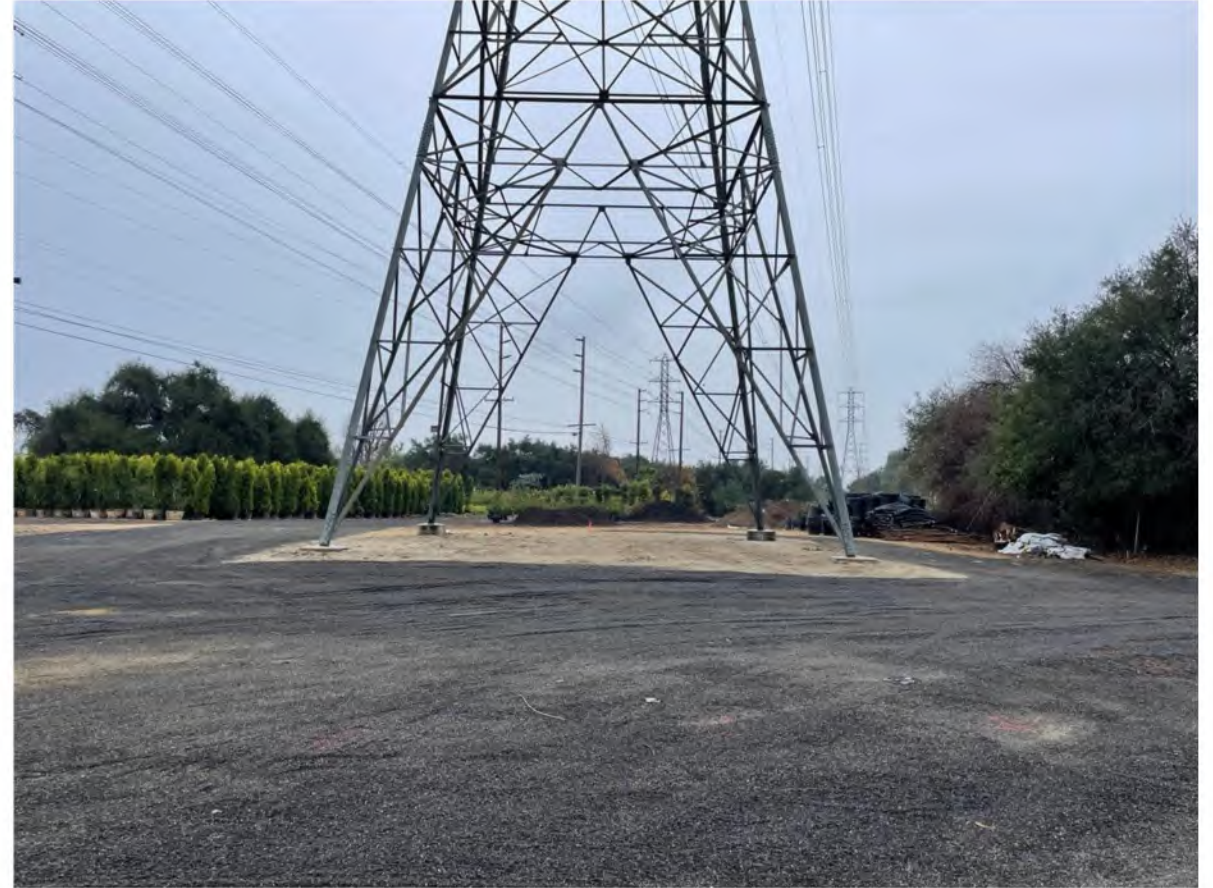
Photo #2. Taken on the eastern portion of the site, western portion of the nursery. Facing south.
