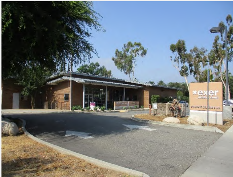
Photograph 12. The east and primary (north) elevations of 3160 East Del Mar Boulevard, looking southwest.
