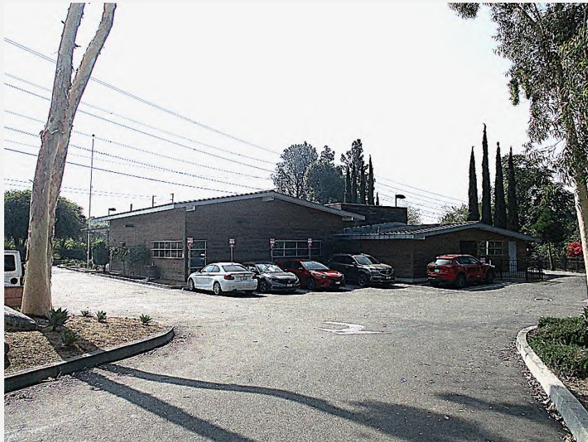
Photograph 15. The primary and west elevations of 3160 East Del Mar Boulevard, looking southeast.
