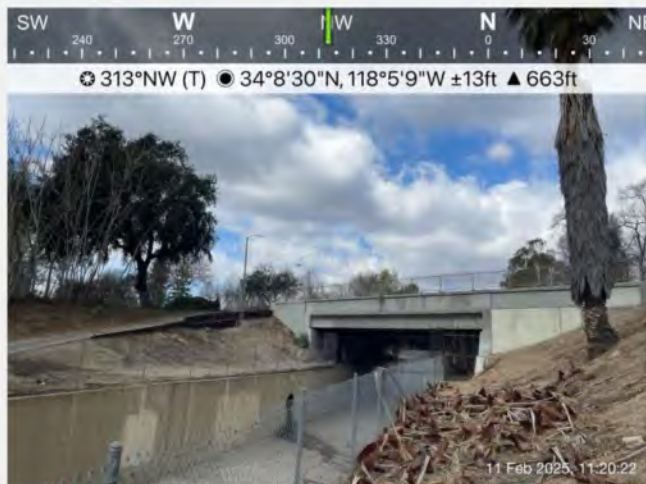
Photo 1. View of Del Mar Blvd spanning Eaton Wash in the northern area of the project site.
