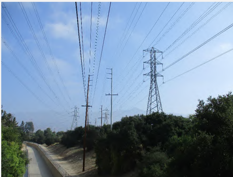
Photograph 2. The SCE Mesa-Anita-Eaton Transmission Line along the Eaton Wash Channel, looking northeast.
