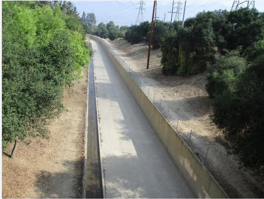
Photograph 3. View of the Eaton Wash Channel, looking north.
