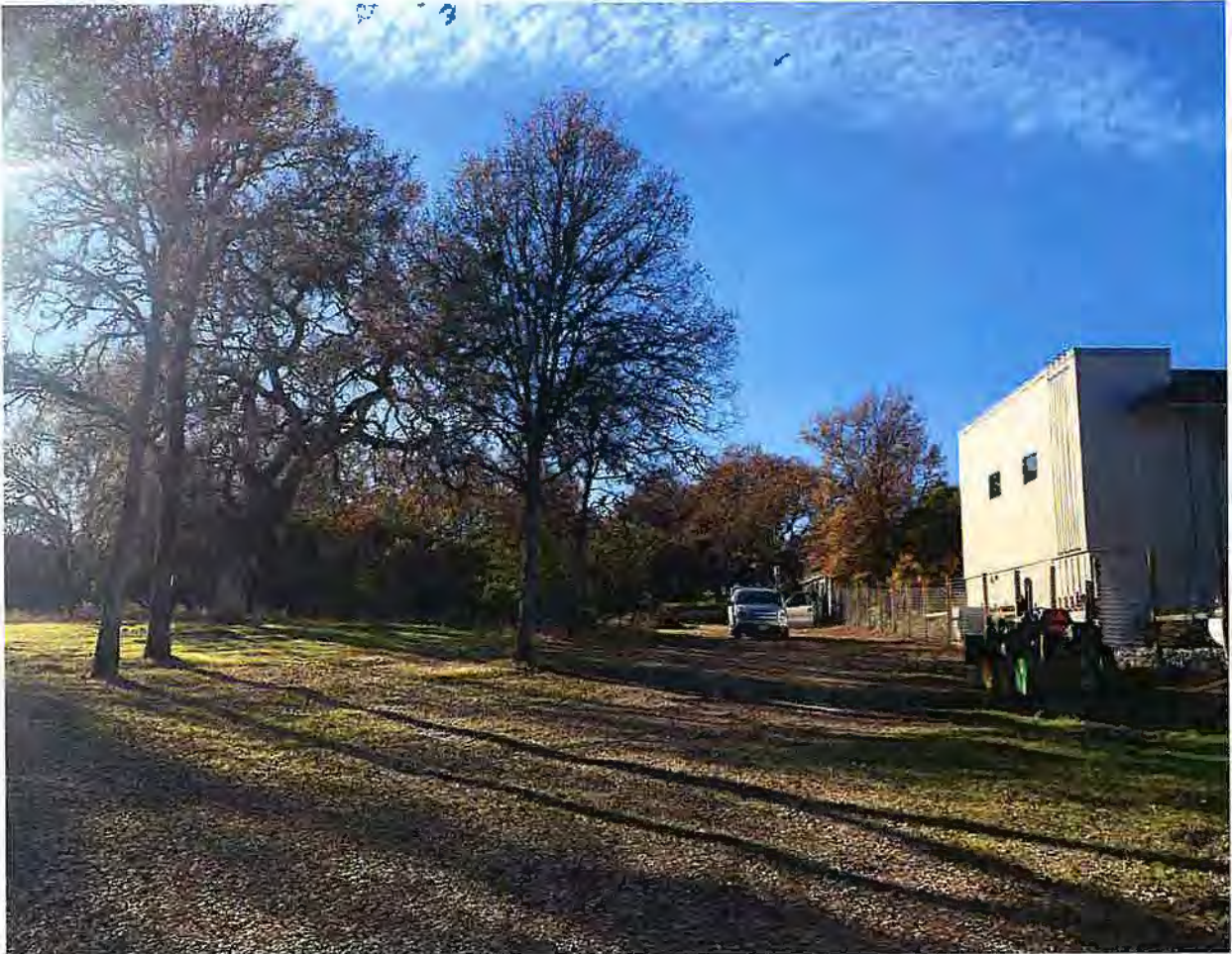
Photo 5. Another view (west) with trees #43, #44 and #29 pictured near existing and proposed road construction. TPZ and 5RZ impacts are expected.
