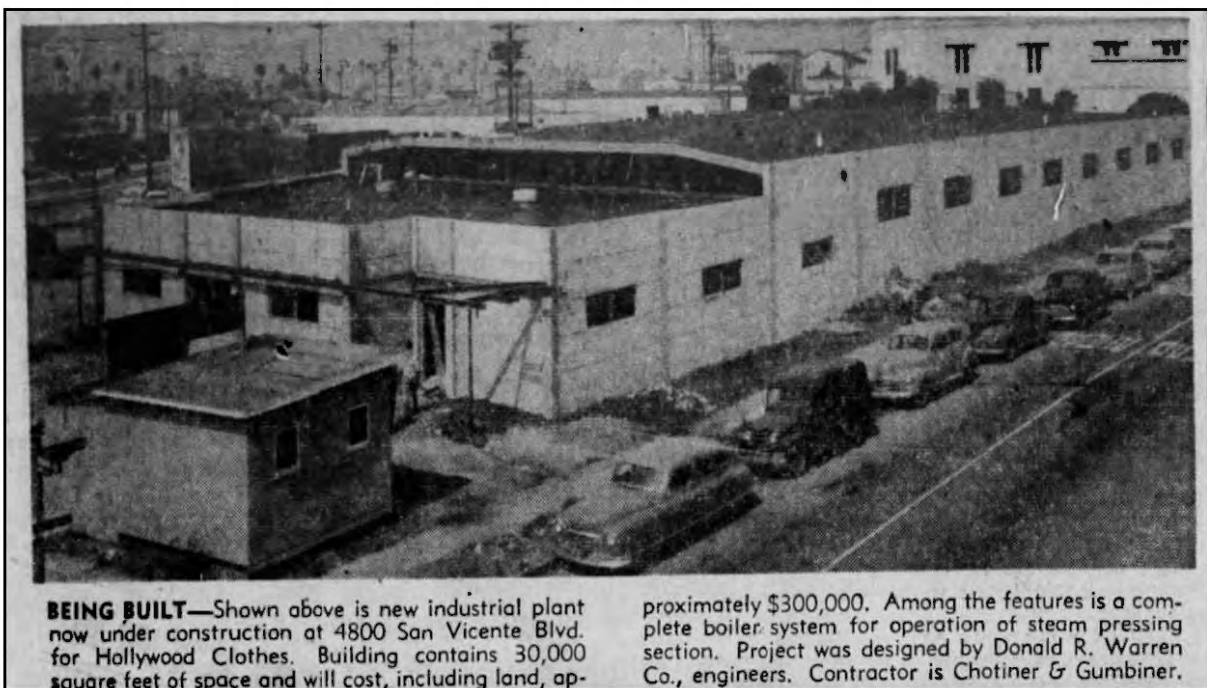
Figure 3. Hollywood Clothes Under Construction, 1956 (LAT 10 June 1956:154)
