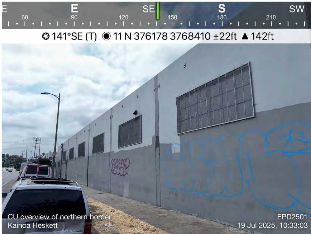
Photo 4: Overview of Project Site from Central Portion of N Boundary
