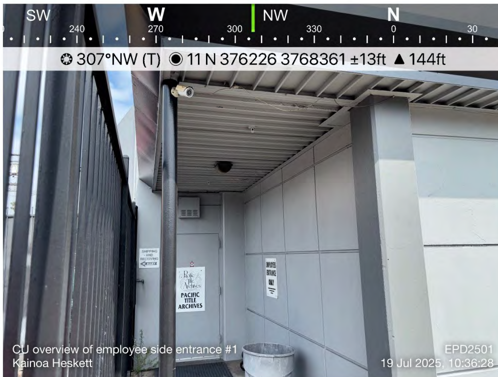
Photo 6: Overview of S Side of E Elevation of 4800 San Vicente Building
