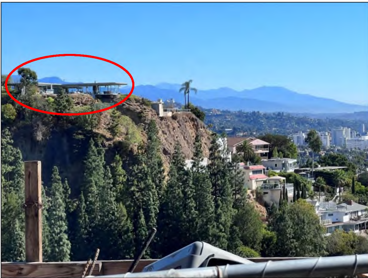
Figure 10. Profile view of Stahl House and Marlay Drive below including the concrete retaining wall at 1509 Marlay Drive and the residence at 1521 Marlay Drive, view to east
