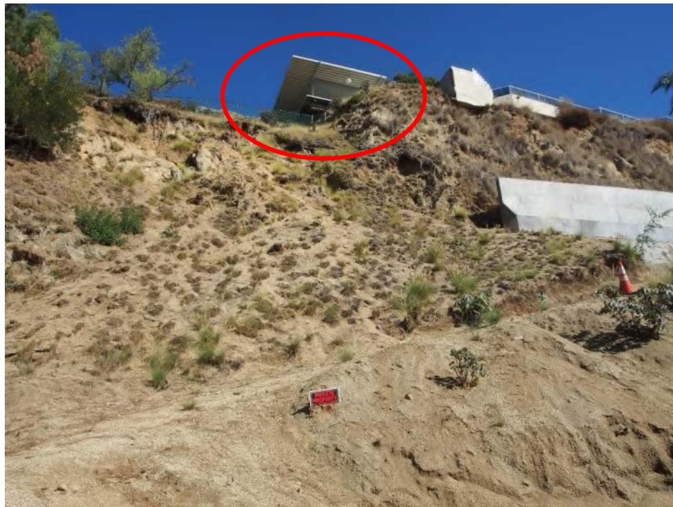
Closer view looking up at the Stahl House (circled in red) from N. Marlay Drive, facing north
