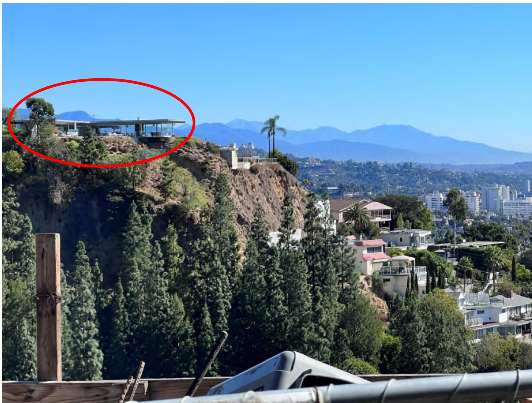
Profile view of Stahl House and Marlay Drive below including the concrete retaining wall at 1509 Marlay Drive and the residence at 1521 Marlay Drive, view to east
