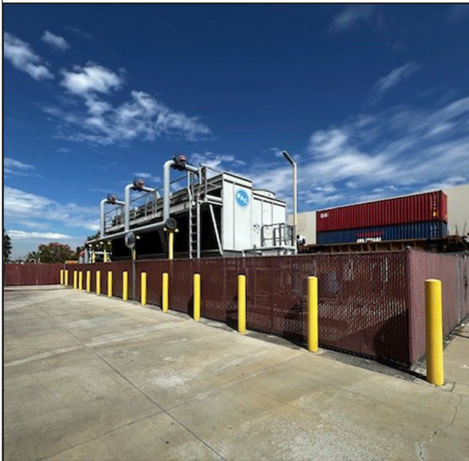
Photo 5 shows interior parking lot facing northeast.
