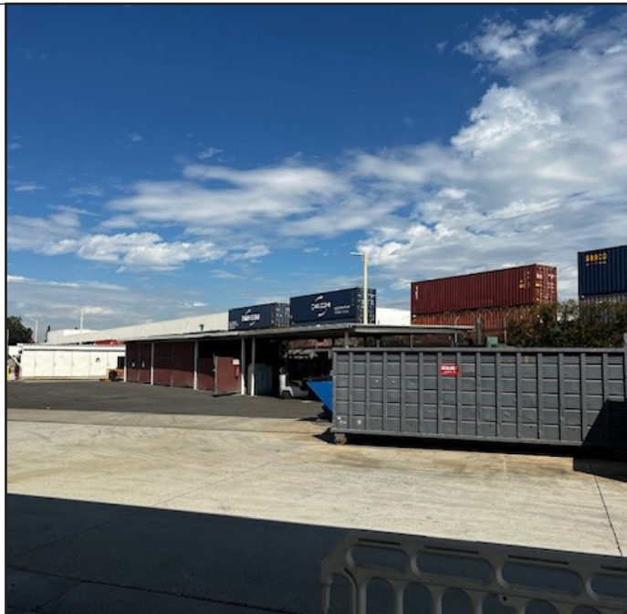
Photo 4 shows interior parking lot facing east.
