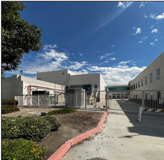
Photo 6 shows driveway facing east from Beach Boulevard.
