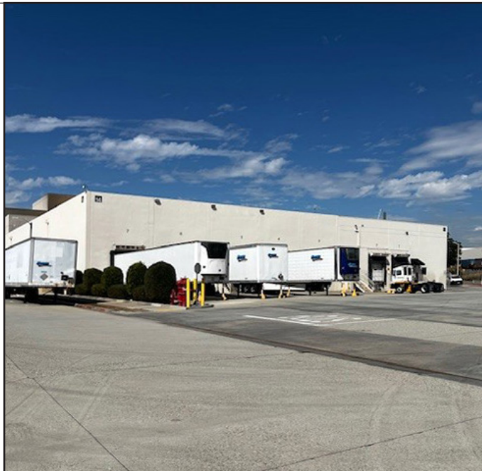
Photo 3 shows interior parking lot facing northwest.
