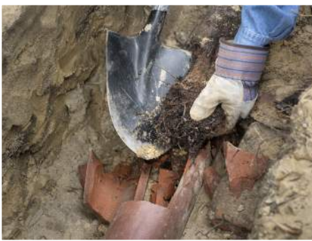
Plumber making repairs on private lateral
