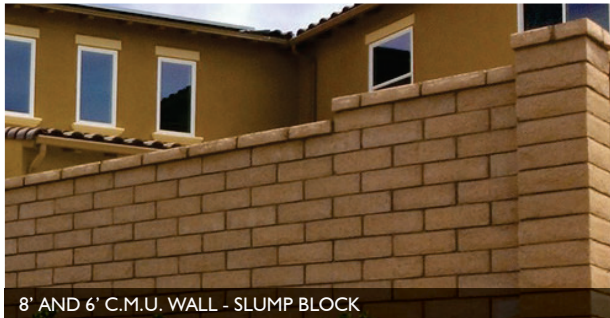
8' AND 6' C.M.U. WALL - SLUMP BLOCK
