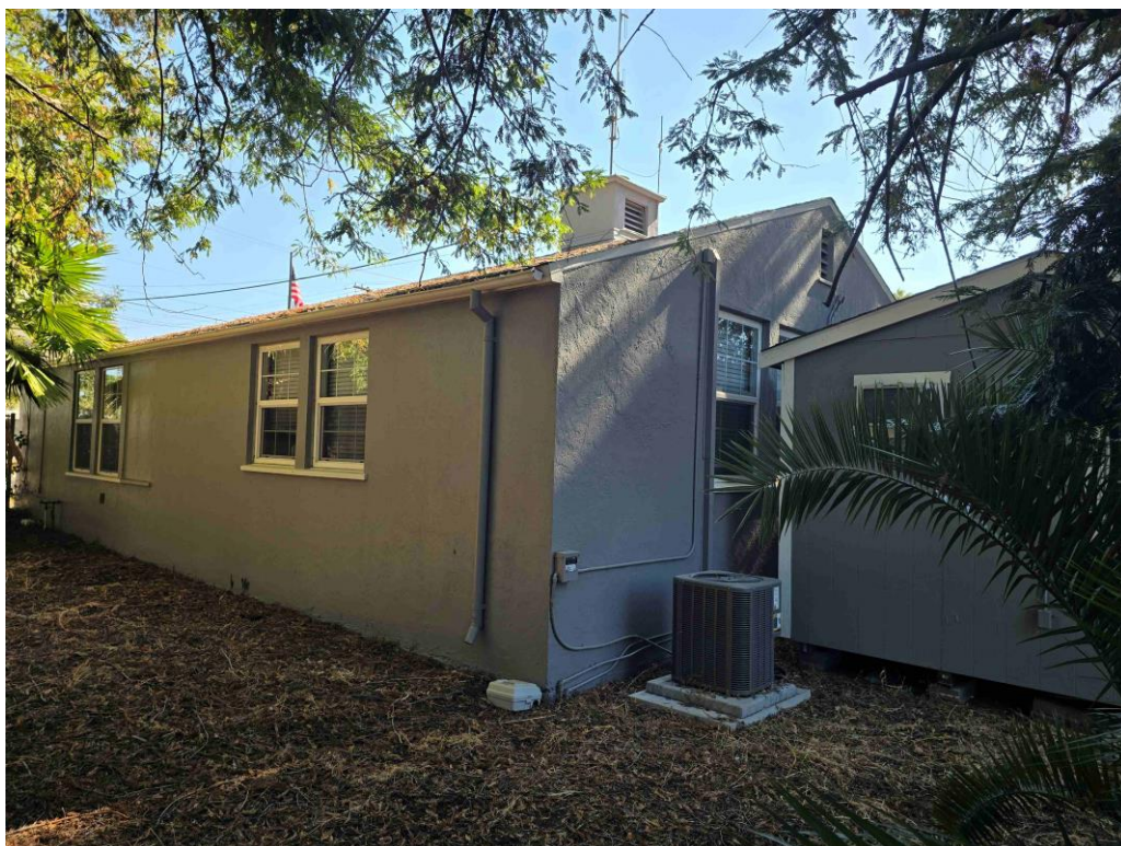
Plate 4. Photograph of West elevation, facing northeast, taken 8/8/24. Note the replacement hung windows and one infilled window (date/s of modifications unknown).
