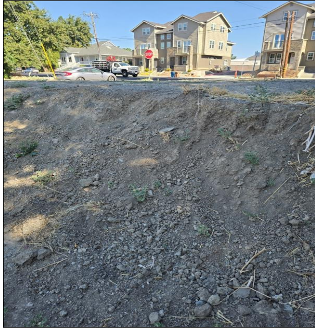
Photograph 3 – Close-up view of soil pad located in western portion of project site, taken 7/25/24, facing north by northwest.
