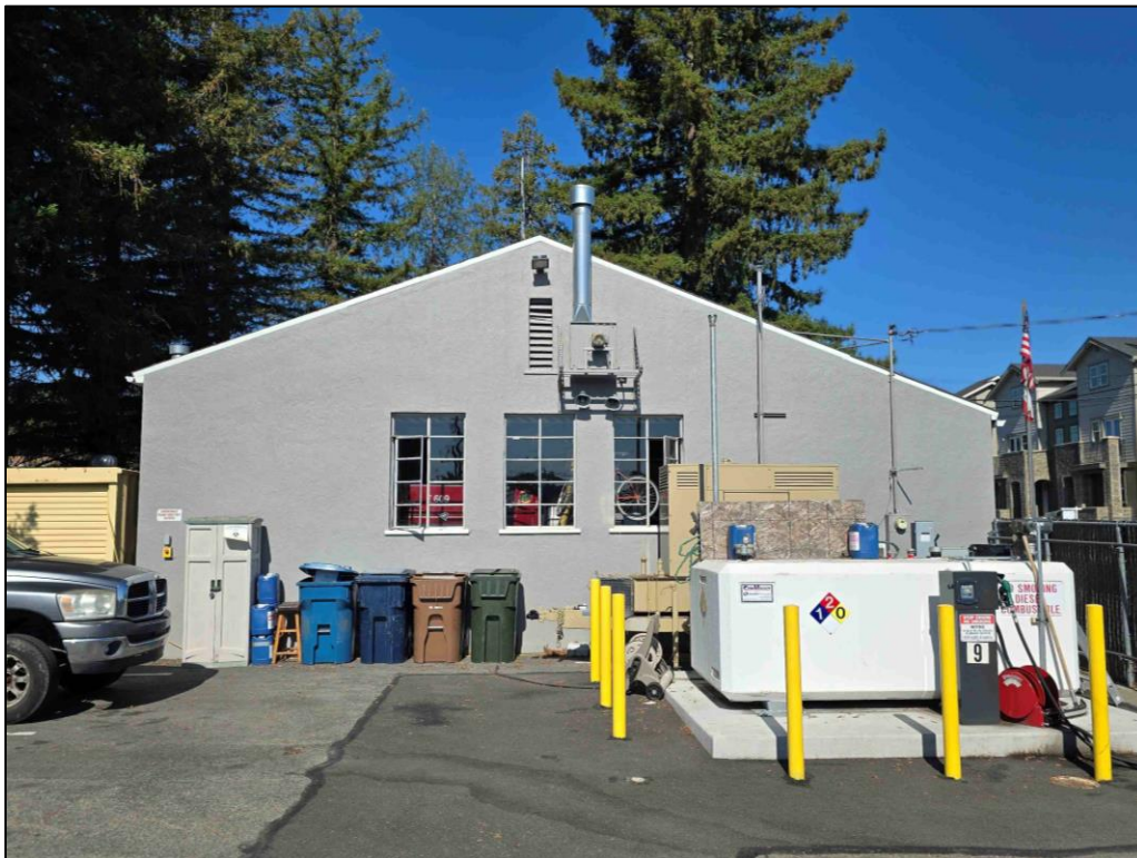
Plate 2. Photograph of Fire Station Building East elevation, facing west, taken 8/8/24.
