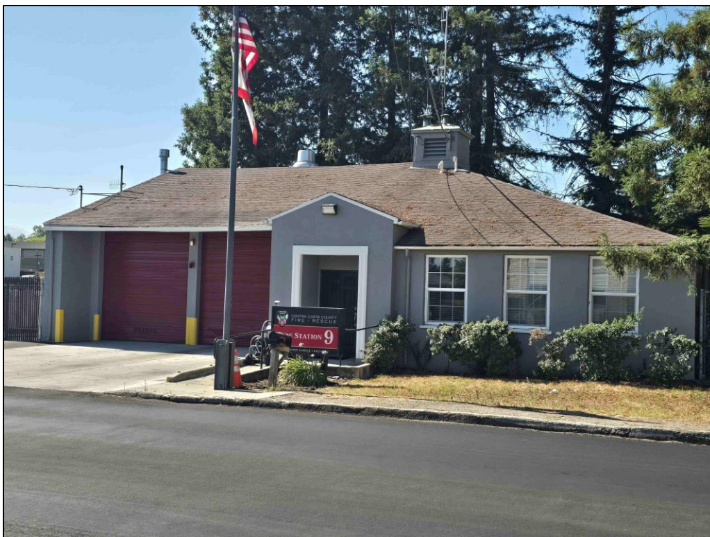
Plate 1. Photograph of North (primary) façade of Fire Station Building, facing south, taken 8/8/24. Note the replacement pedestrian door and windows (date(s) of modifications unknown).
