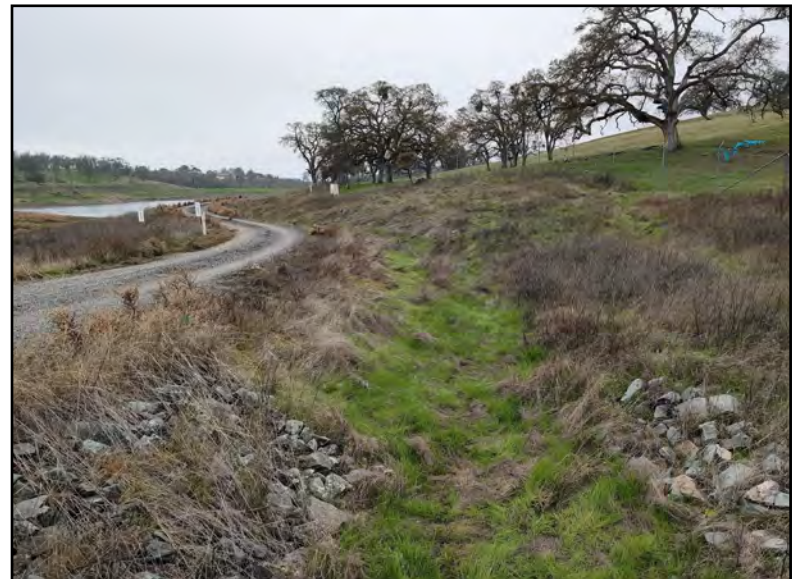
Photo 8. Drainage Ditch (DD-02) along the Roadside of the Lower Effluent Storage Pond (view south; December 16, 2025).
