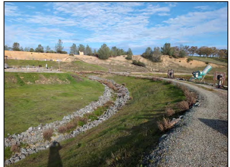
Photo 6. Drainage Ditch (DD-01) within the Facility (view north; December 16, 2025).
