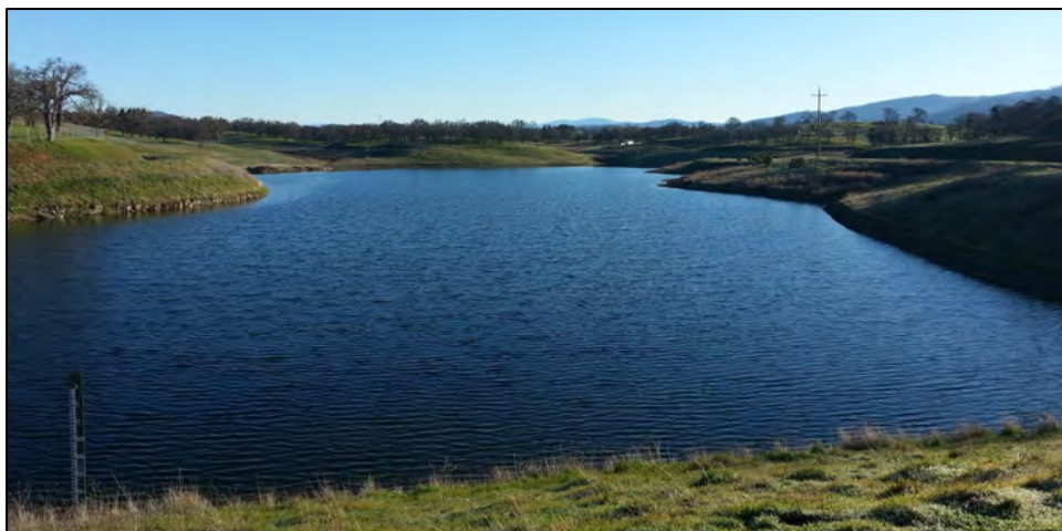
Photo: Lower Effluent Storage Pond (LESP)
