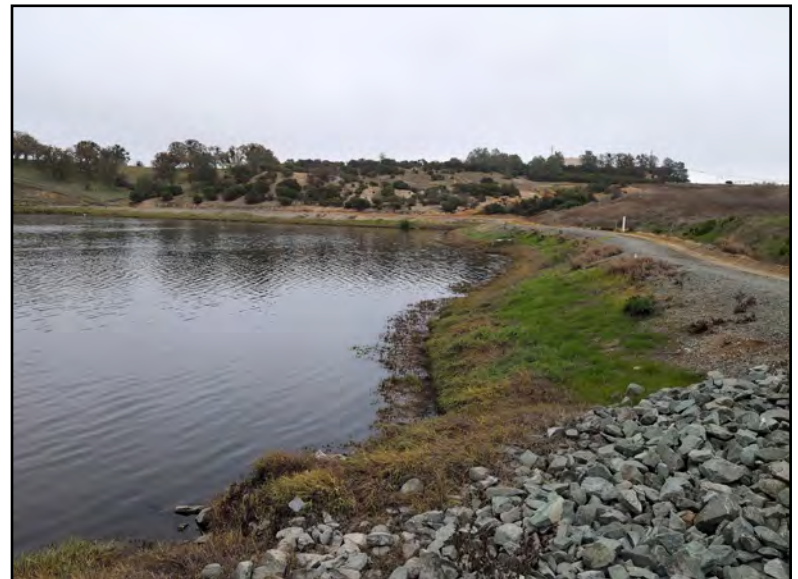
Photo 4. Representative Photo of the Upper Effluent Storage Pond (WTP-02) (view east; December 16, 2025).
