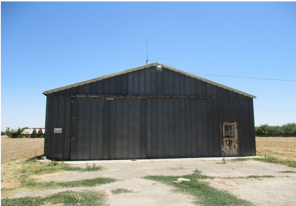
Nondescript storage structure that will presumably be demolished at 24499 Robertson Bl (view east).
