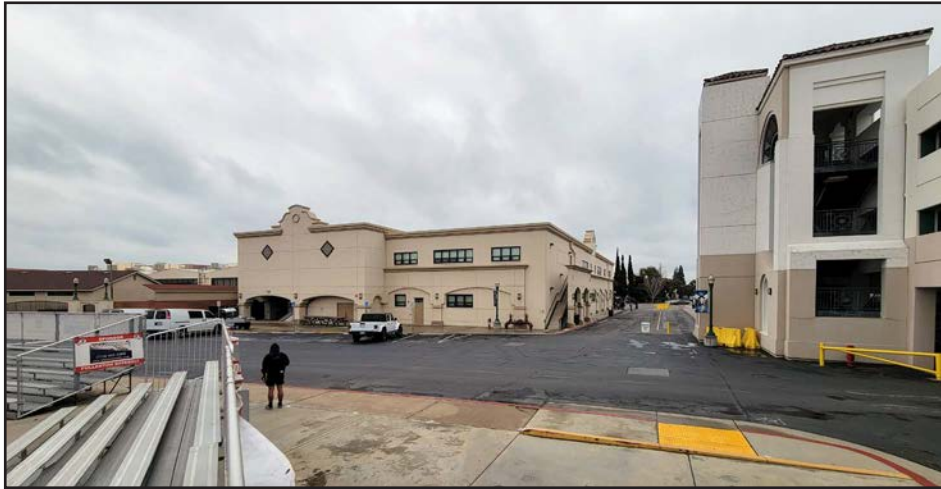
View 11. From the southern end of the baseball field, looking south at the parking structure and educational buildings on the Fullerton College campus surrounding the project site.
