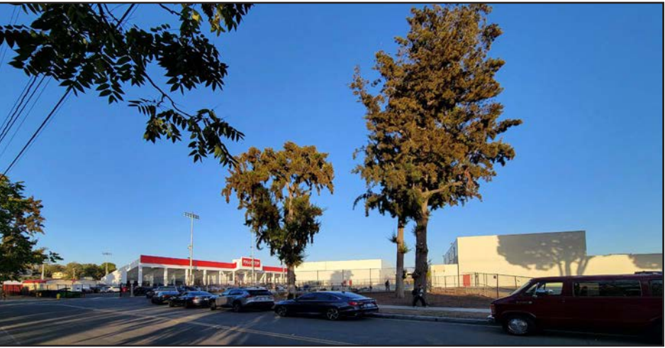
View 9. From the western side of N Pomona Avenue, looking northeast at the tennis courts, northern parking lot, and landscaped area on the project site.
