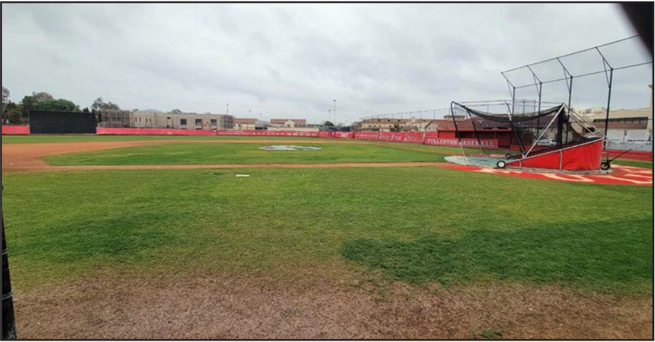
View 5. From the western end of the baseball field, looking east at the baseball field and the surrounding fencing on project site.
