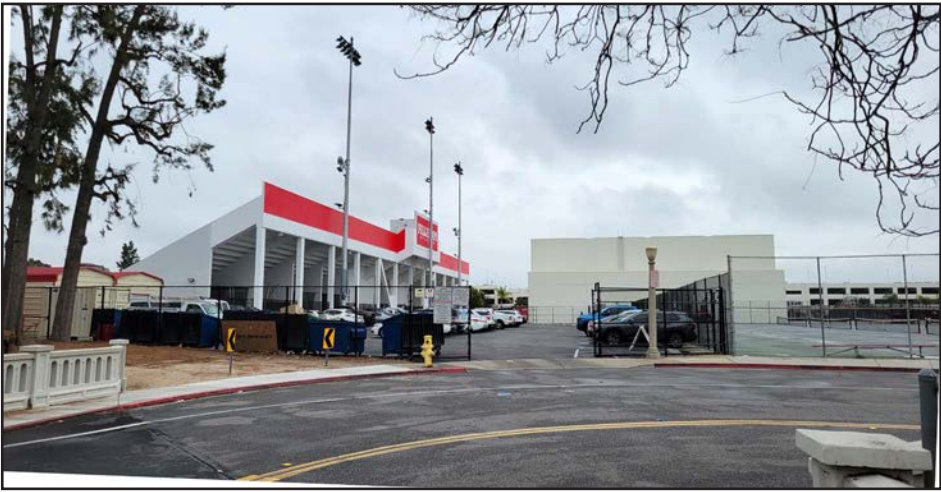
View 8. From the eastern end of E Glenwood Avenue, looking east at the northern parking lot and tennis courts on the project site.
