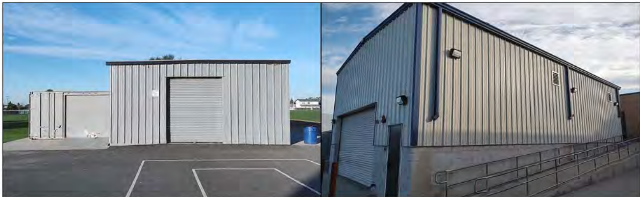
Steel outbuildings. Left : grounds maintenance building, view to the north; right : outbuilding against main building mass, view to the northeast
