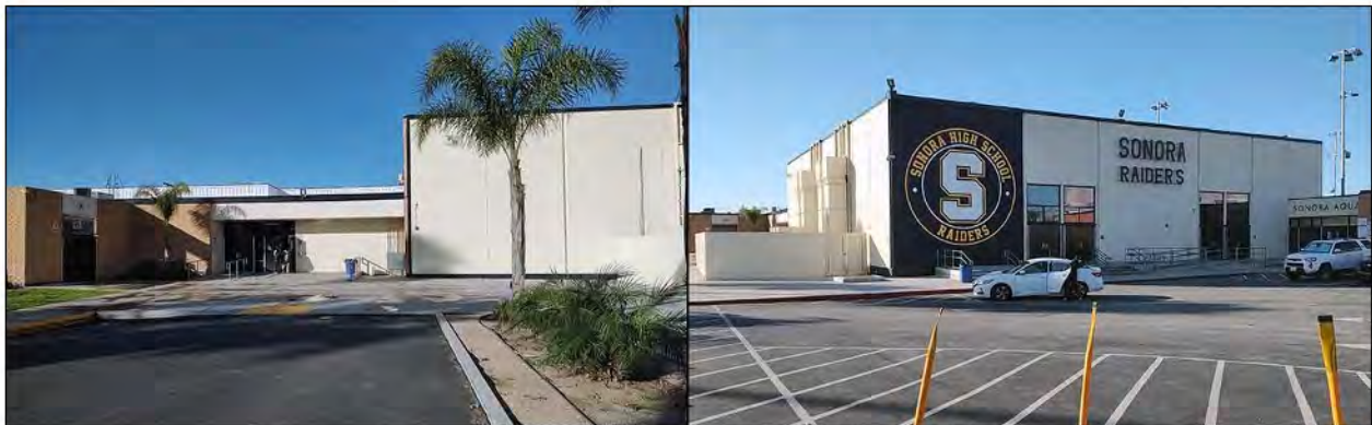
Gym. Left: connection between the main building and the gym, view to the west; right: northern façade of the gym, view to the south
