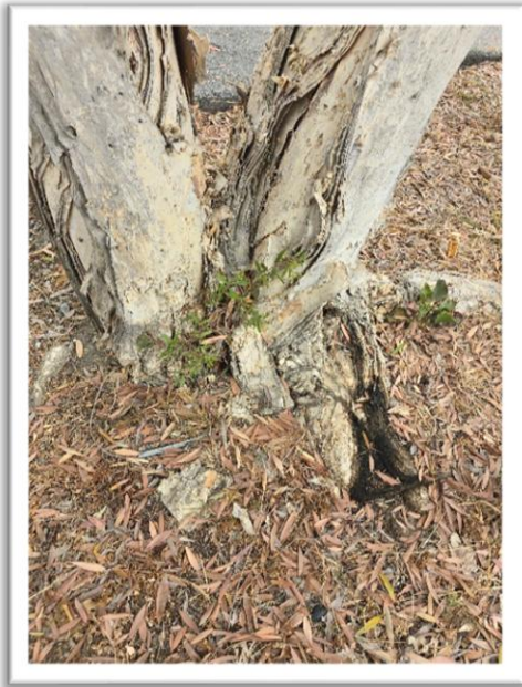
Plate 9. This is a view of decay on a structural root (#792).
