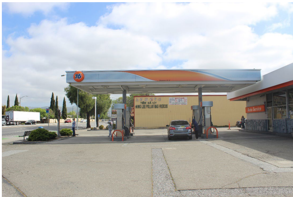
Photograph 7: 1152 Tully Road fueling terminal with eight gas pumps, camera facing northeast, April 23, 2025.
