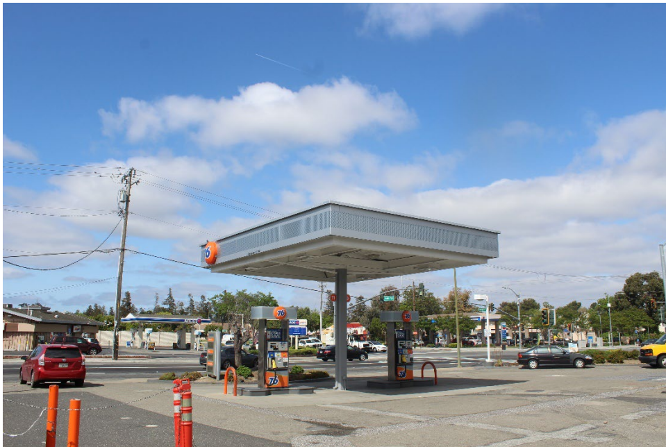
Photograph 6: 1152 Tully Road fueling terminal with four gas pumps, camera facing northwest, April 23, 2025.
