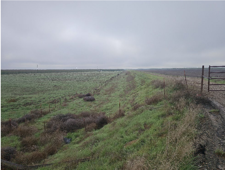
Photo 2. Grassland at the bypass levee. Photo facing south.
