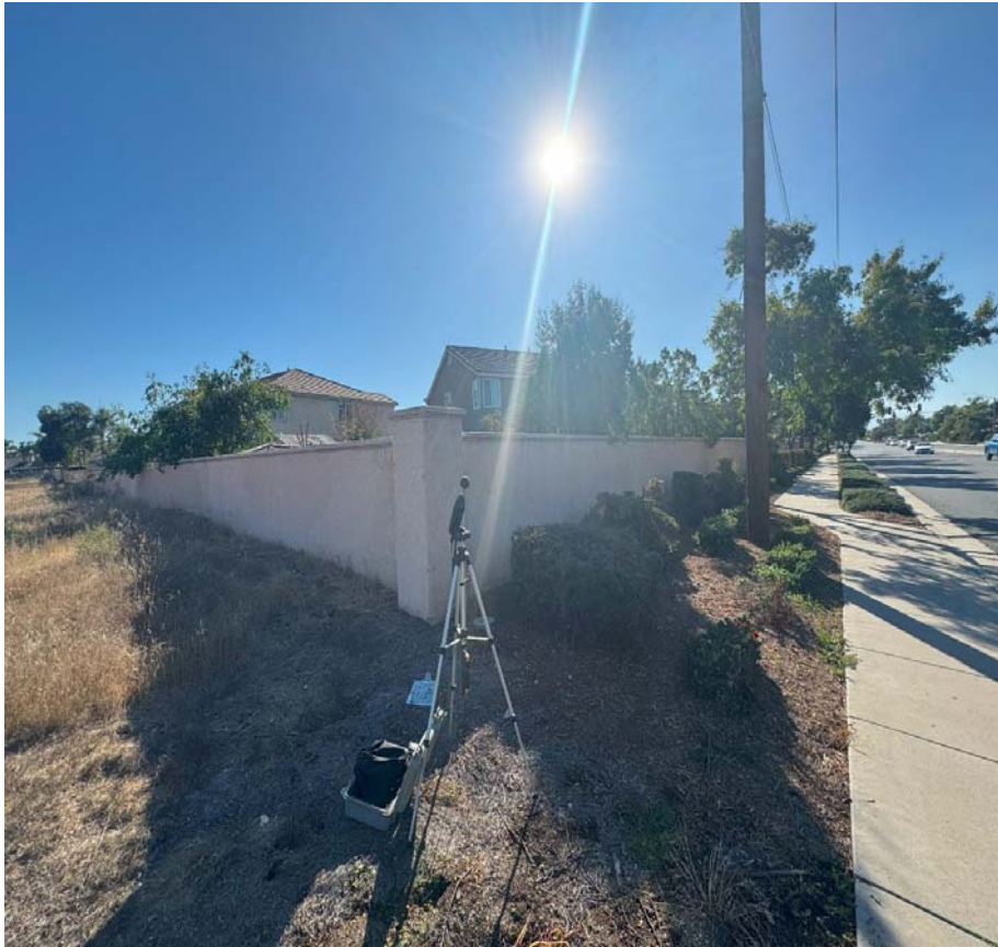
NM1 looking towards backyard of residence 28760 Ave Marbella, Menifee ( behind 6' tall concrete block & stucco wall ) Newport Road heading W on the right.
