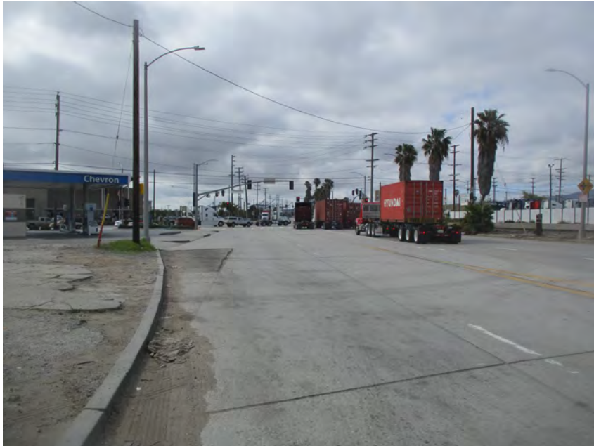
View of south end of Alameda Street looking south.
