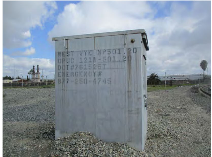
Concrete vault on Wilmington Wye.
