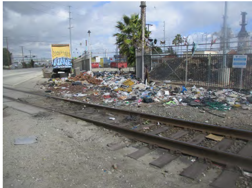
Dumped trash at north end of Wilmington Wye.
