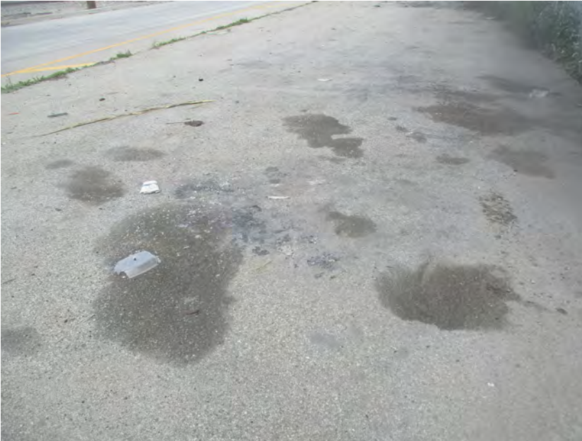
Oil stained asphalt on east contiguous sidewalk at 1100 Alameda St.
