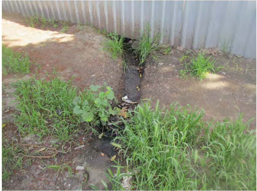
Run-off onto unpaved sidewalk west of 1262 Alameda.
