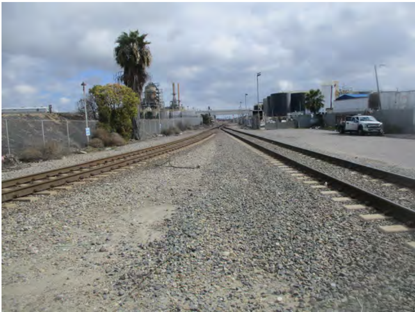
East junction of Wilmington Wye, Valero Tank Farm on the left.
