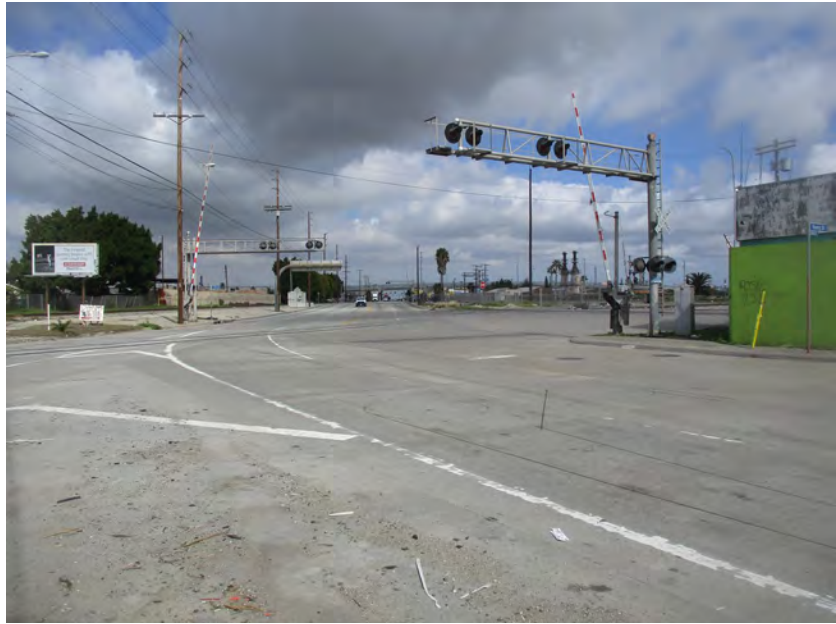
Railroad crossing at Alameda and Young Streets.
