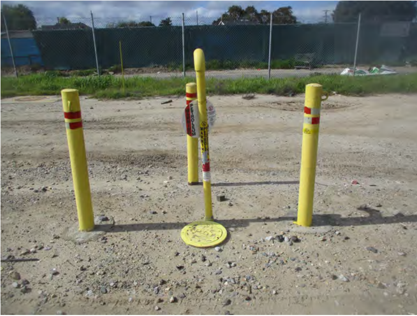
Typical warning markers designating petroleum pipelines.
