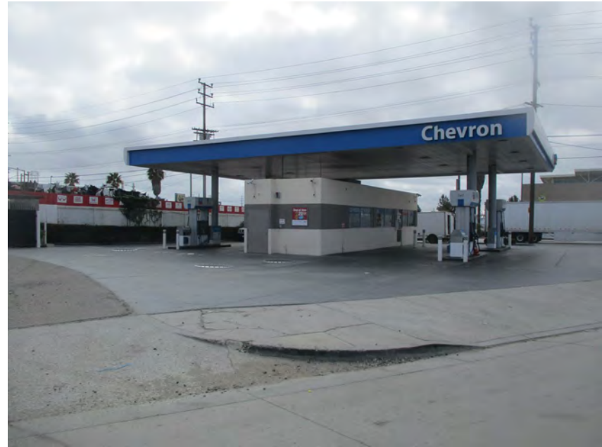
East contiguous Chevron station at Alameda and E. Anaheim.
