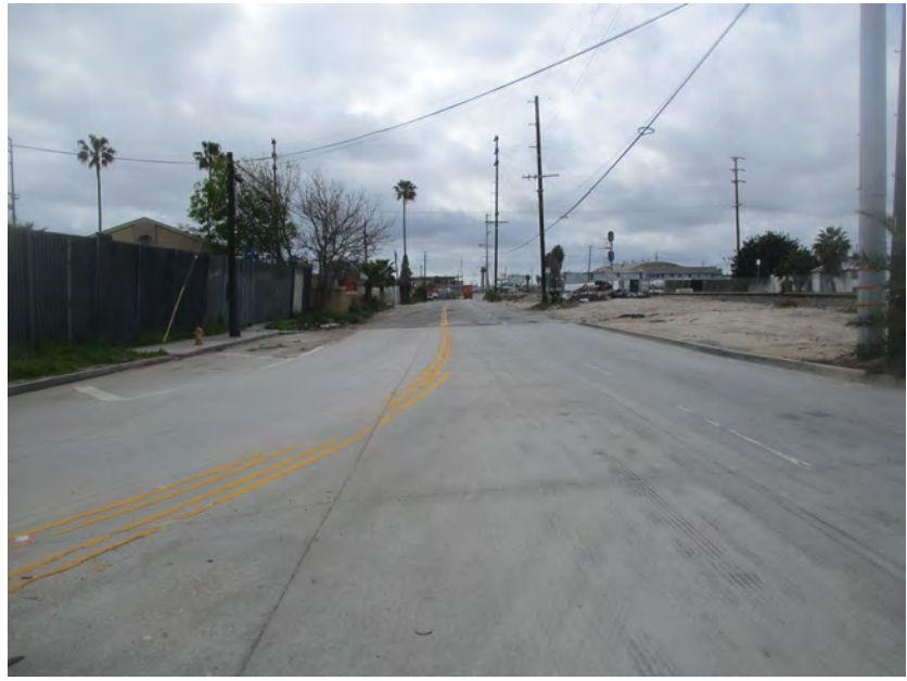
Concrete and asphalt paved Alameda Street looking south
