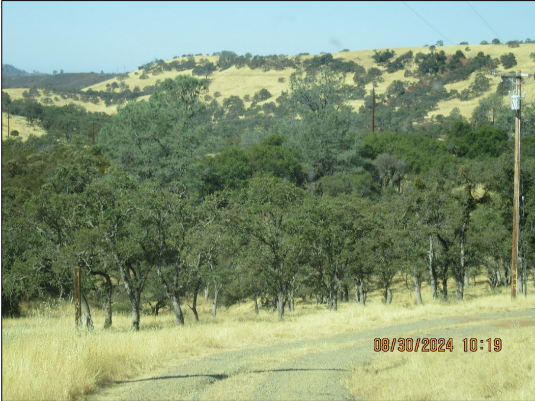
Figure 8: View of power lines on proposed Parcel 4
