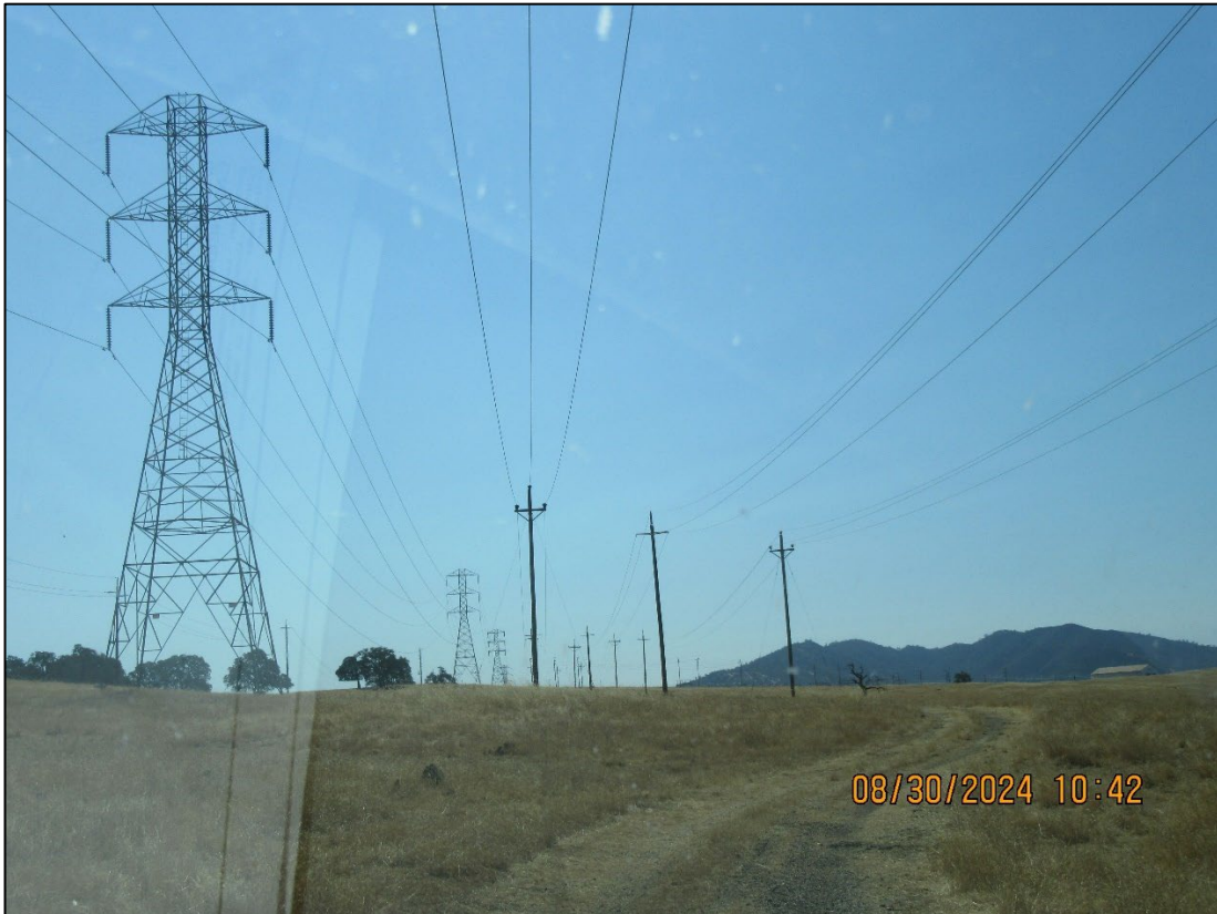
Figure 9: View of road at drainage crossing in proposed Parcel 4
