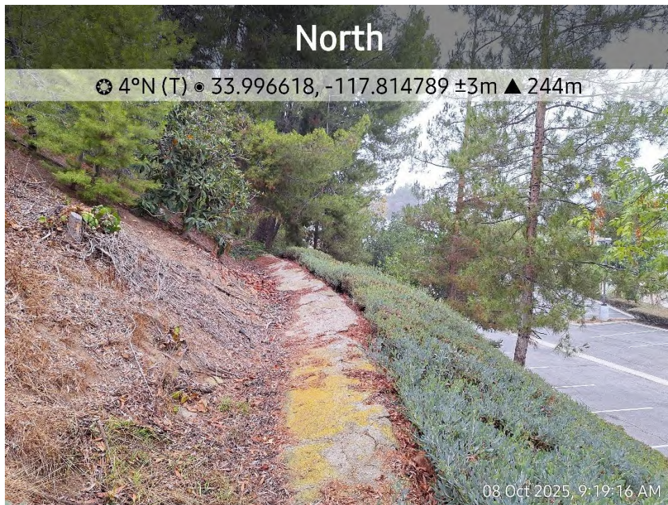
Photograph 8. View of a drainage swale in western hillside.
