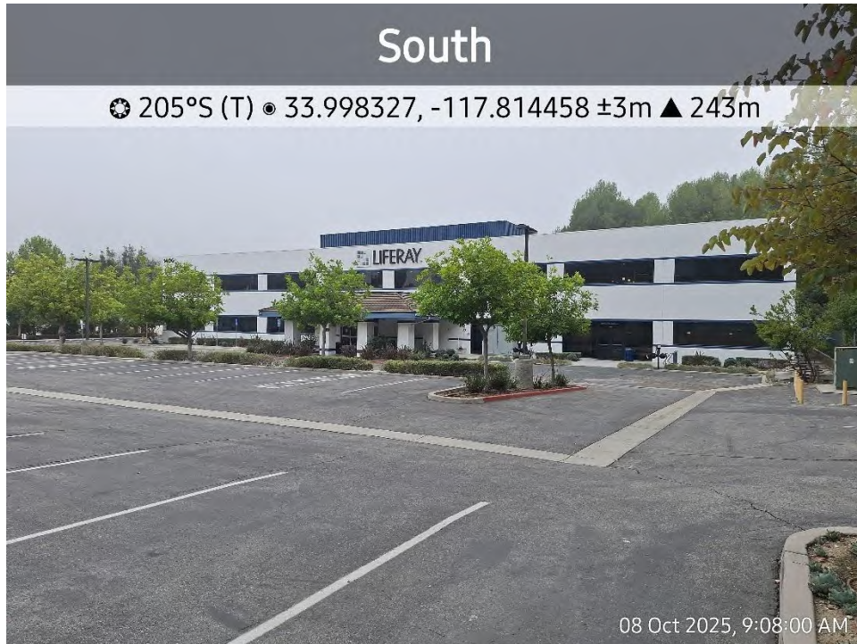
Photograph 1. Overview of project site and northern elevation of office building.
