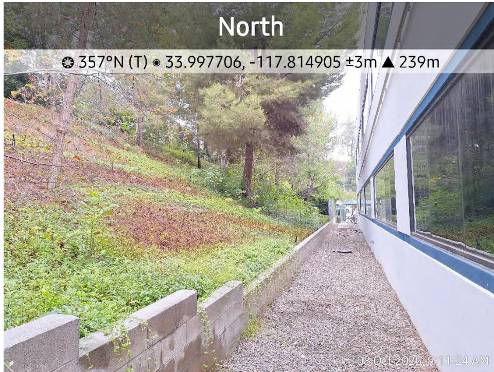
Photograph 5. View along western side of office building and western boundary of the project site.
