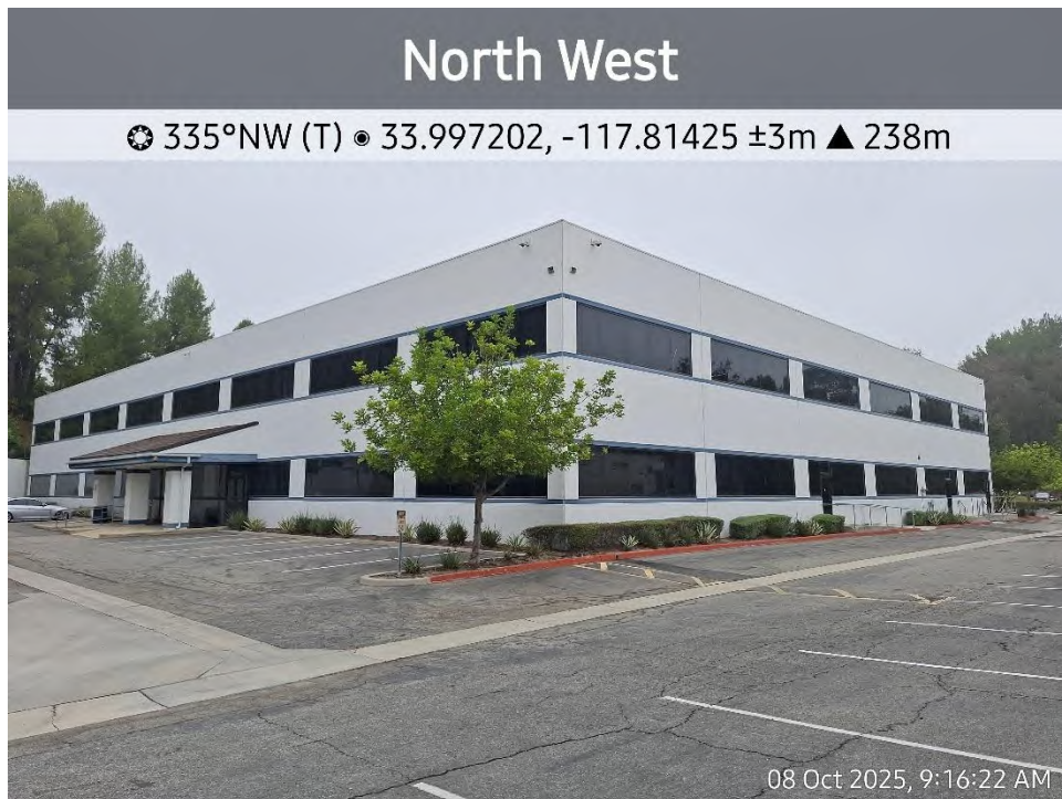
Photograph 2. Overview of southern and eastern elevations office building.
