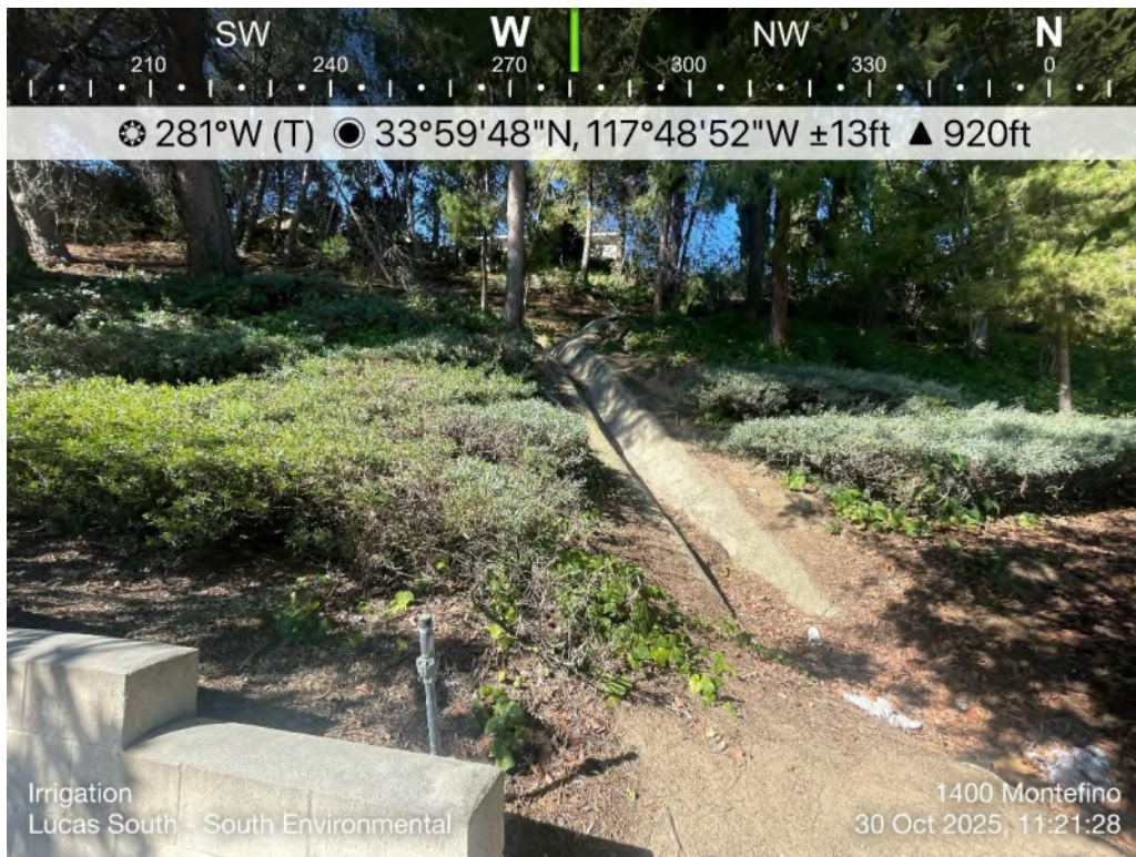
Image 9.) View of concrete channelized drainage and irrigation in the ornamental woodland, facing west.
