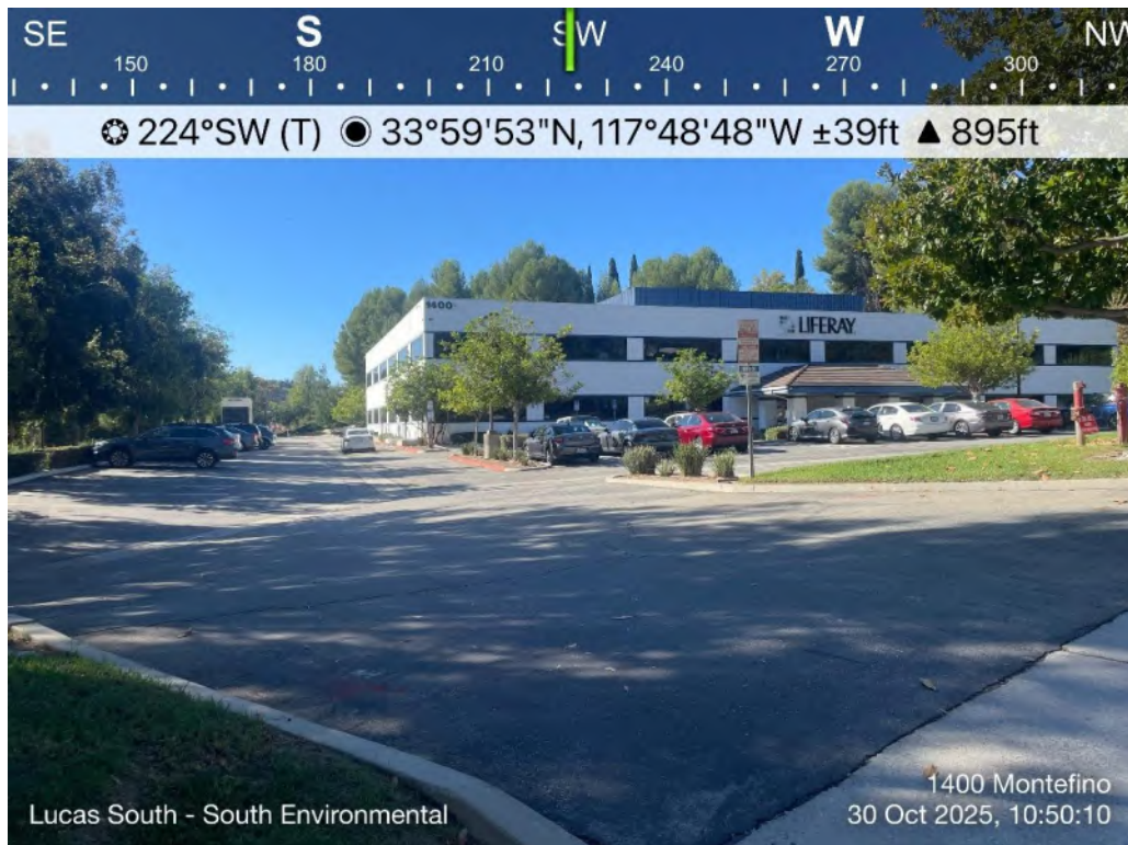
Image 1.) View of 1400 Montefino Ave. commercial development with surrounding ornamental landscaping, facing southwest.
