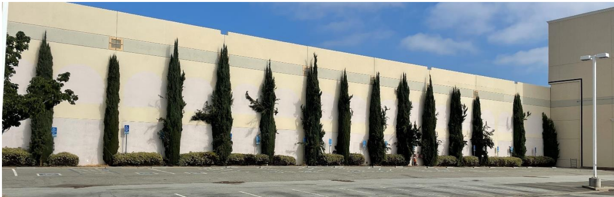
Photo 9. Photo above shows one line of Italian Cypress along the building. Most of the trees have stems that are falling away from the canopies and, if retained, require pruning/shearing work. All trees are considered Protected. However, measurements were not possible at 4.5'.
