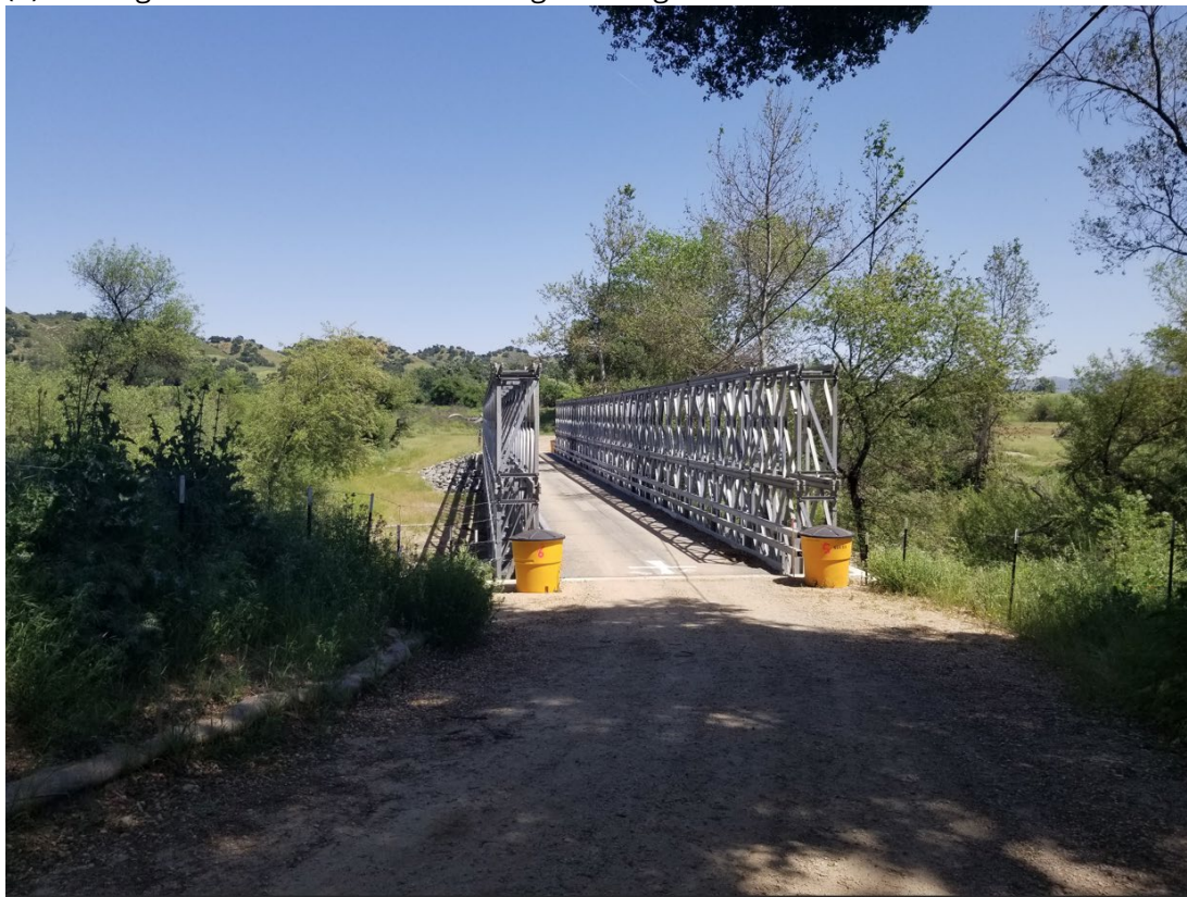
(c) Existing Huasna Townsite Road Bridge looking east.
