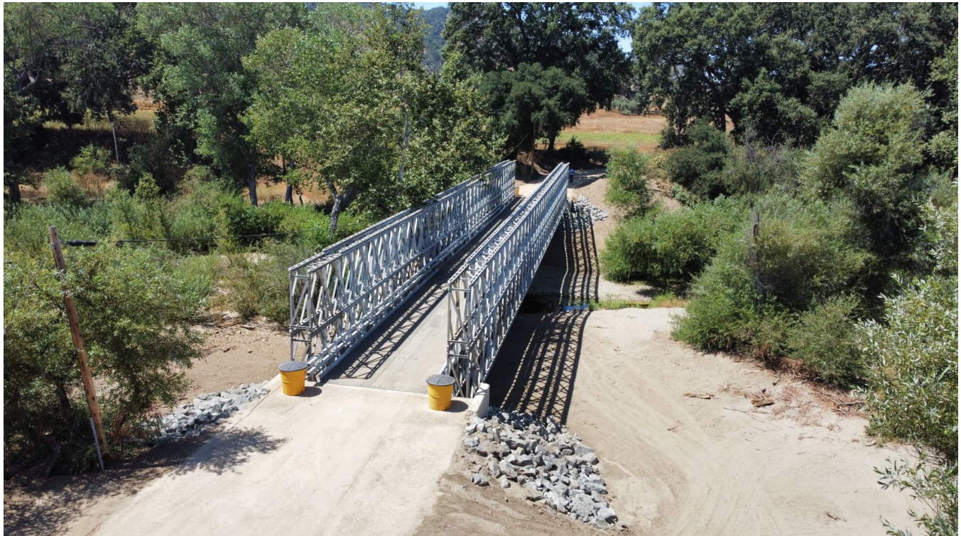
(b) Existing Huasna Townsite Road Bridge looking west.
