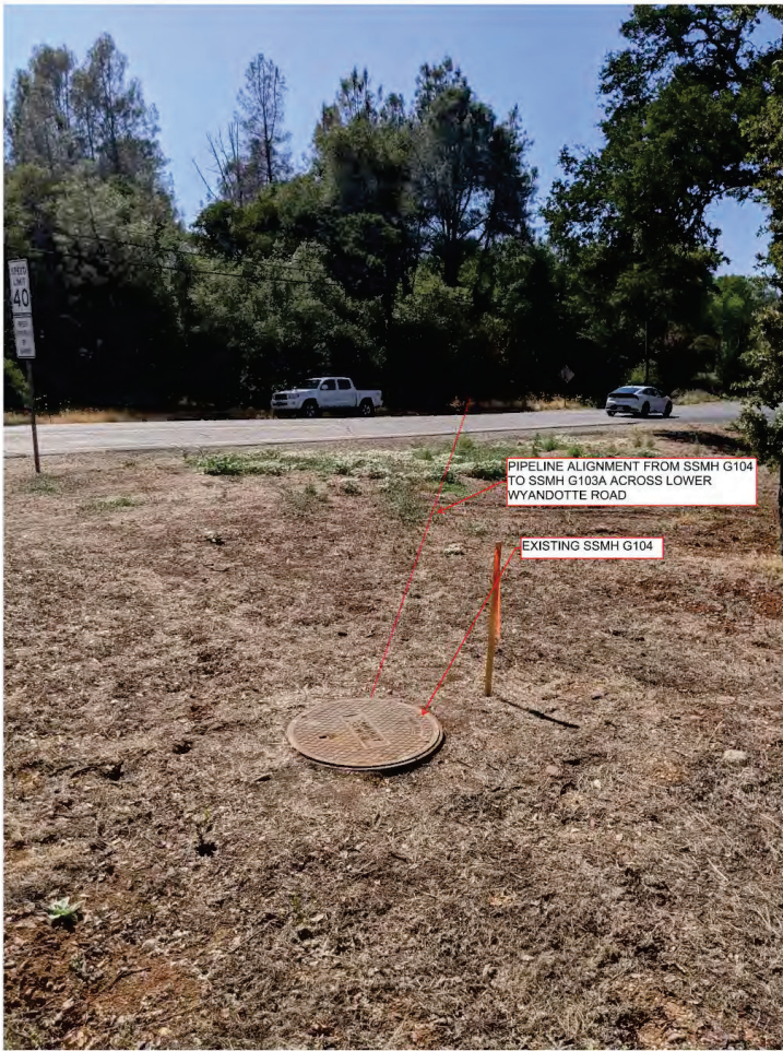
Figure 3: Upstream End of Pipeline Replacement SSMH G104 to SSMH G103A
