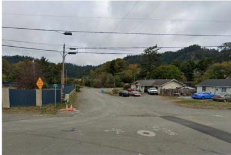
Figure 2-2. Southern Work Area, Facing North
