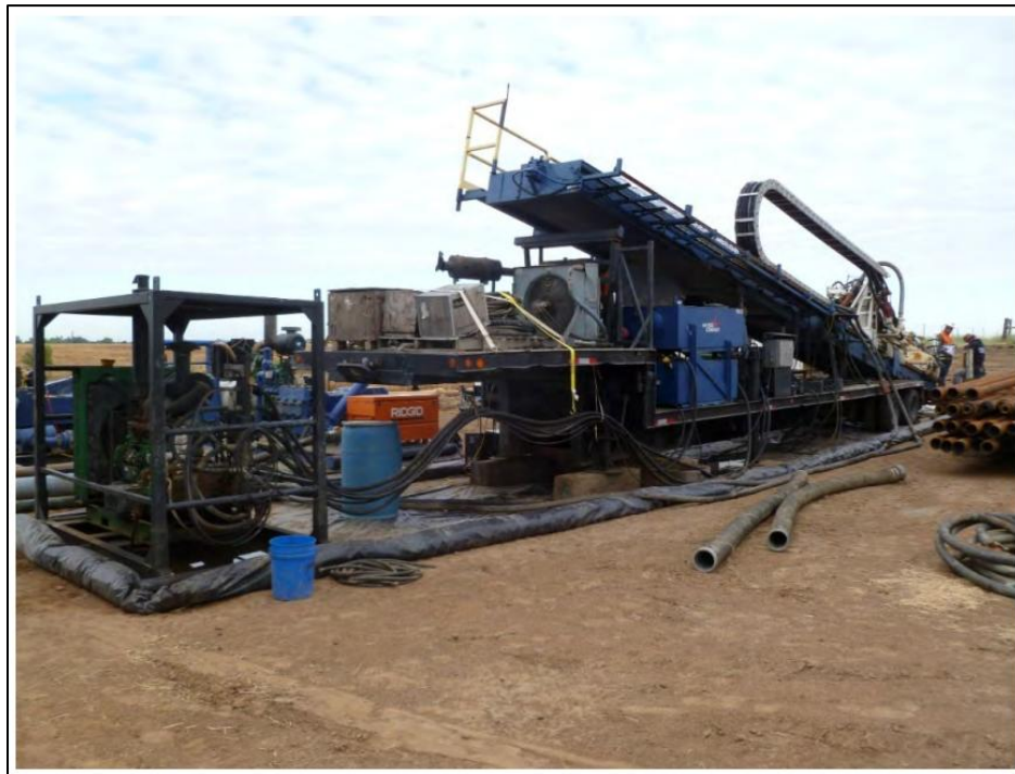
Figure 2-7. HDD Drill Rig
