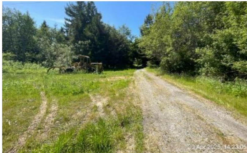
Figure 2-4. Northern Work Area, Facing West
