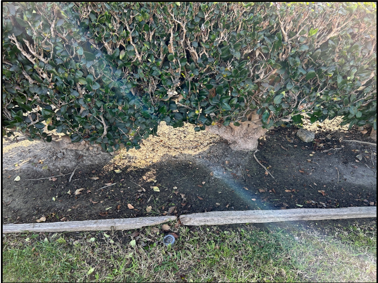
Figure 4.3-8 GROUND SURFACE BELOW HEDGE, NORTH BOUNDARY LANDCAPE BED; VIEW TO THE SOUTH
