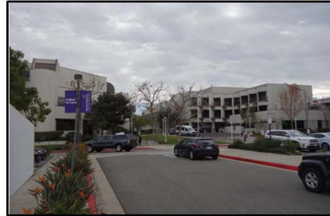
PHOTO 2: View east of the project site looking at three-story medical buildings.
