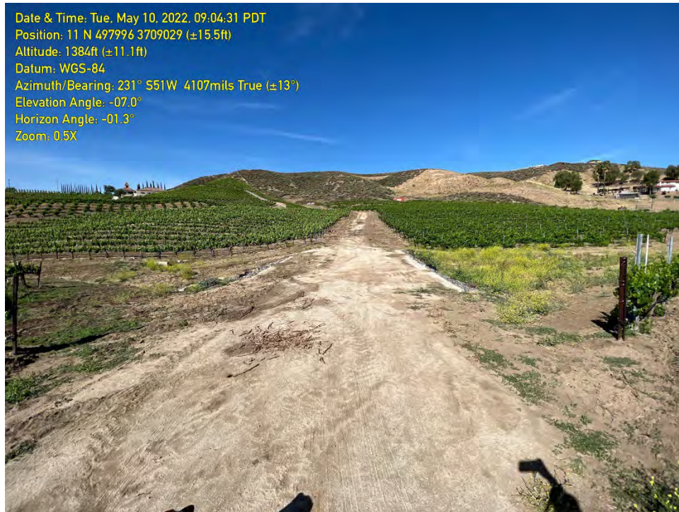
PHOTO 5: The onsite culvert in Feature A at a dirt road crossing.
