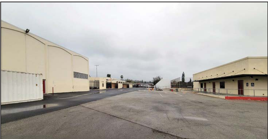
View 12. From the north end of the track and field, looking north at the gymnasium, classrooms buildings, tennis and handball courts, and a vehicle access drive-isle surrounding the project site.
