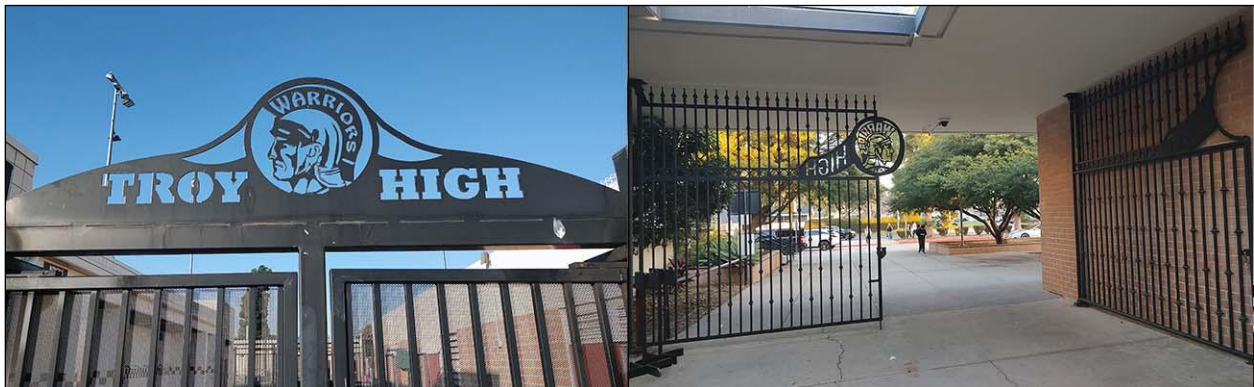
Iron gate elements. Left : pool entrance, view to the west; right : breezeway along office, view to the north
