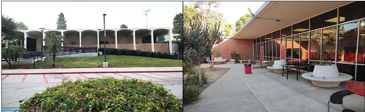
200 Building (Theater and Library). Left : theater front, view to the south; right : west side of Library, view to the northeast
