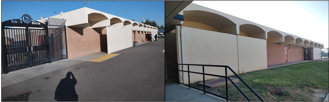
Locker rooms. Left : boys' locker room, view to the northwest; right : girls' locker room, view to the southeast
