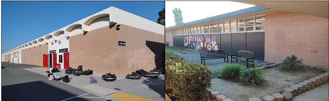
400 Building. Left : southeast corner, view to the northwest; right : north side, view to the southeast
