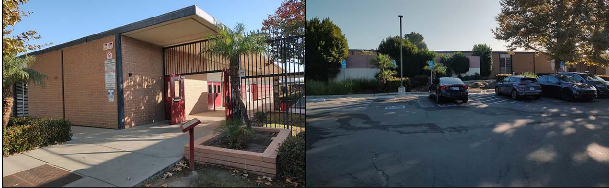
300 Building. Left : southwest corner, view to the northeast; right : modern utility additions, view to the east
