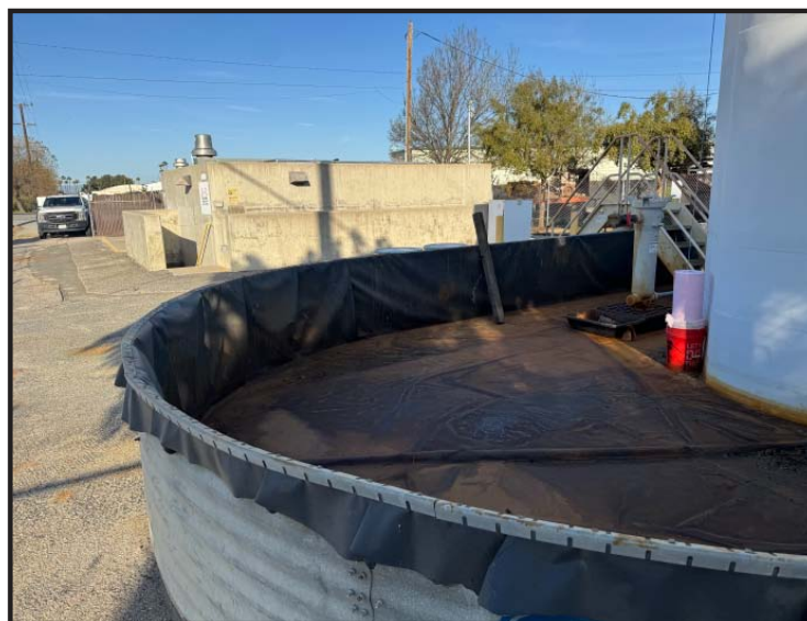
PHOTOGRAPH 6 - Project Site 1, EMWD Cawston Lift Station - L3121
