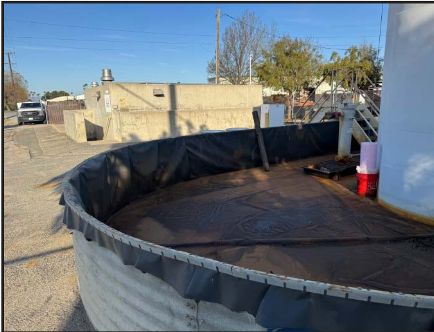
PHOTOGRAPH 6 - Project Site 1, EMWD Cawston Lift Station - L3121
