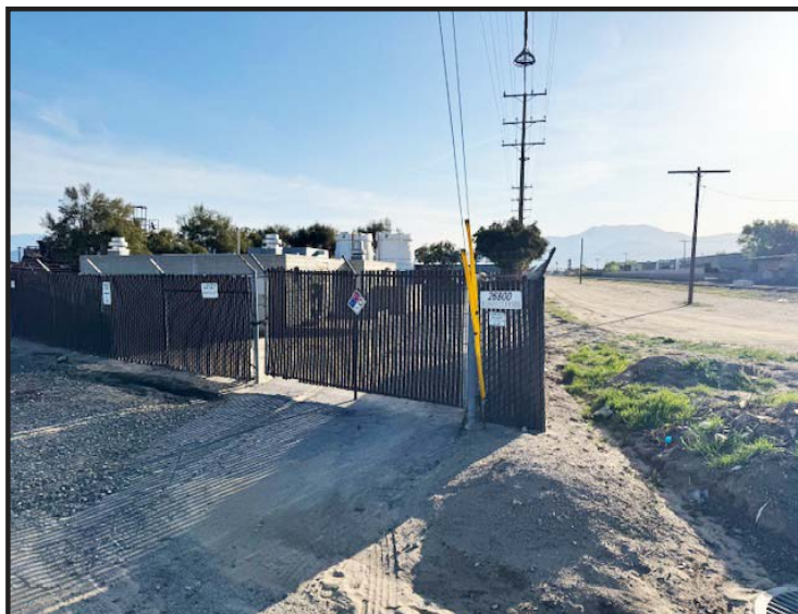
PHOTOGRAPH 5 - Project Site 1, EMWD Cawston Lift Station - L3121
