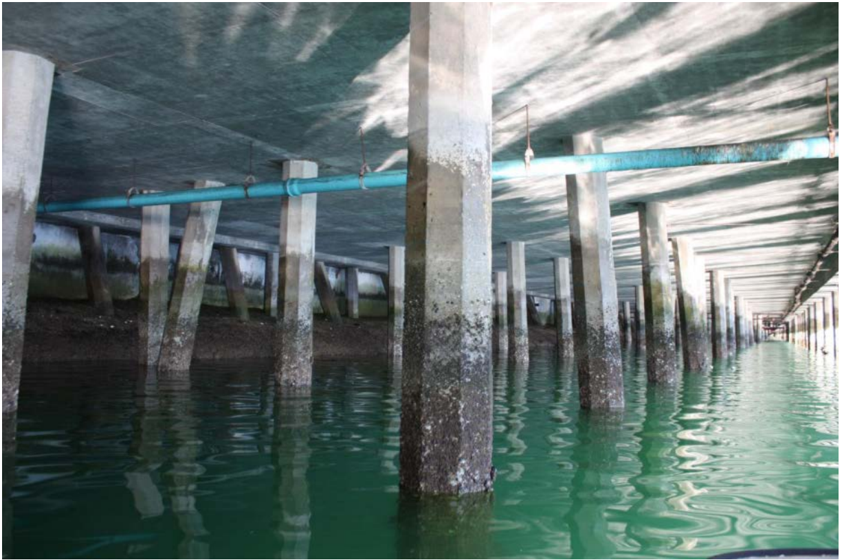
Figure 5 Typical Condition Underneath Wharf 2
