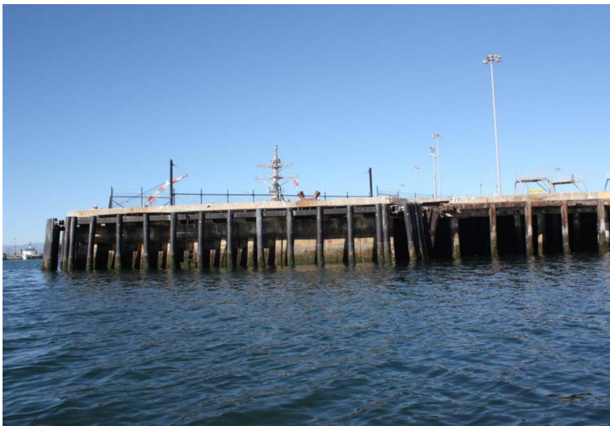
Figure 4 Corner Where Wharf 2, Berth 4 (Right) Meets Wharf 3 (Left)
