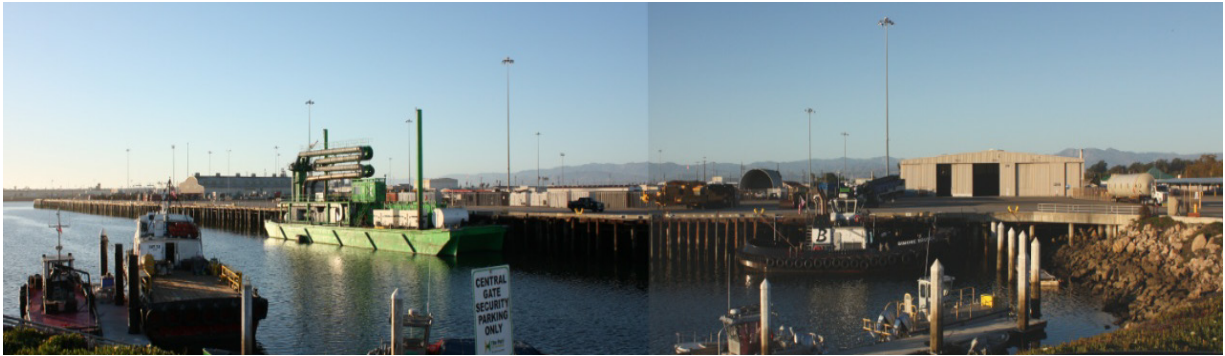
Figure 2 Wharf 2: Berth 4 (Background) and Berth 5 (Foreground)
