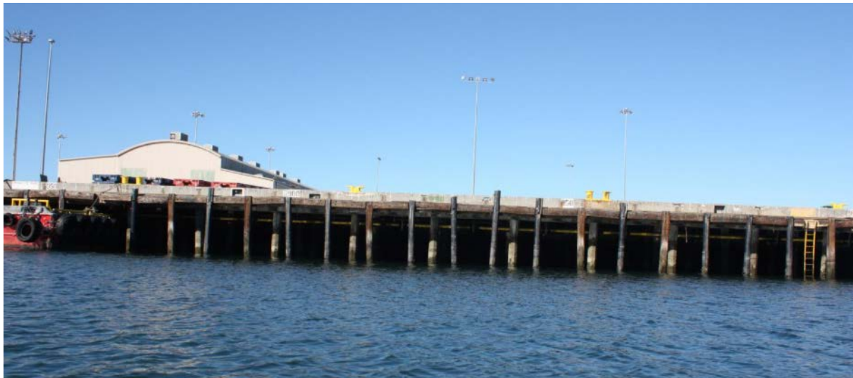
Figure 3 Typical Wharf 2, Berth 4, Fender Pile System
