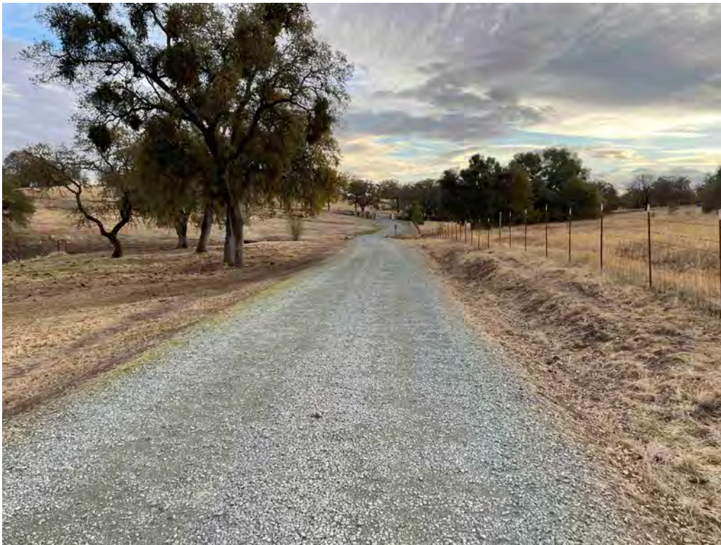
Existing access road to proposed tower site and route of new fiber-optic cable installation. View looking south.
