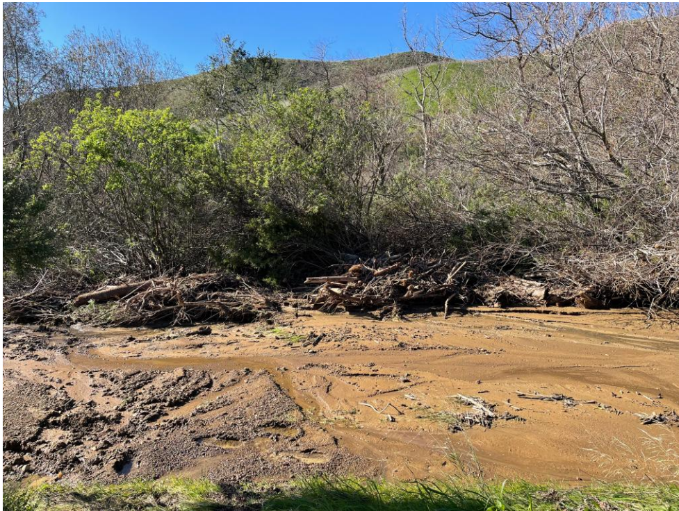
Accumulated debris and silt covering the access road prior to the vehicle bridge at Baron Ranch (January 9, 2026).
