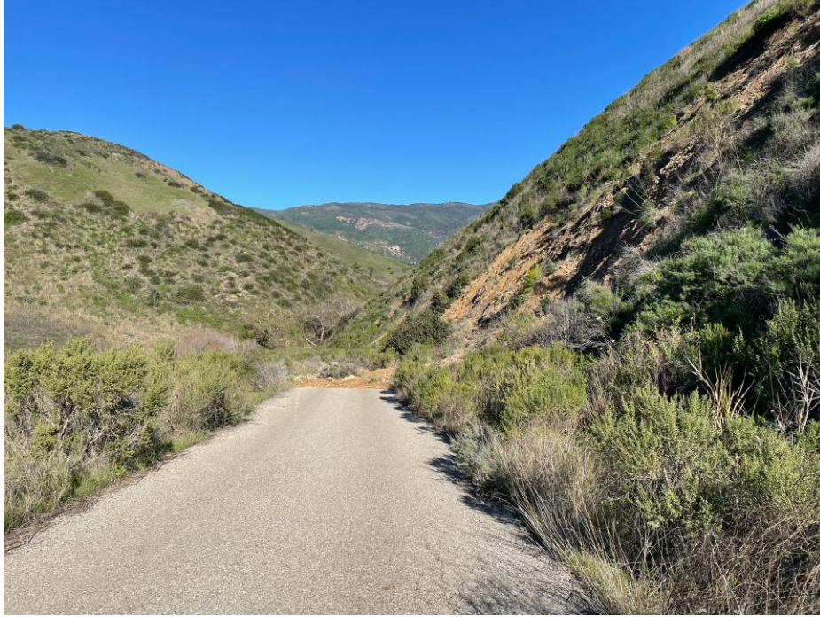
Mudslide crossing roadway with slope failure into Baron Ranch (January 9, 2026).
