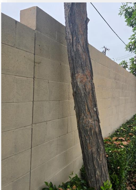
Plate 1. This is a view of a tree planted in close proximity to a block wall (#502).
