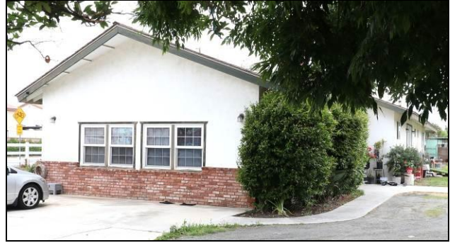
South and east elevations, view northwest (5/6/25).
