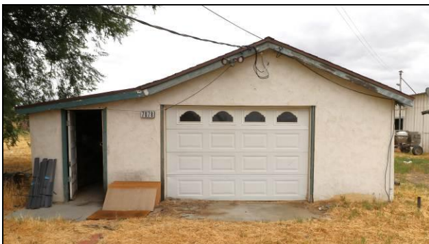
Garage and storage addition, view east (May 6, 2025).
