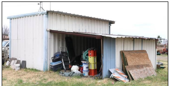
Metal storage shed and addition, view northeast (May 6, 2025).
