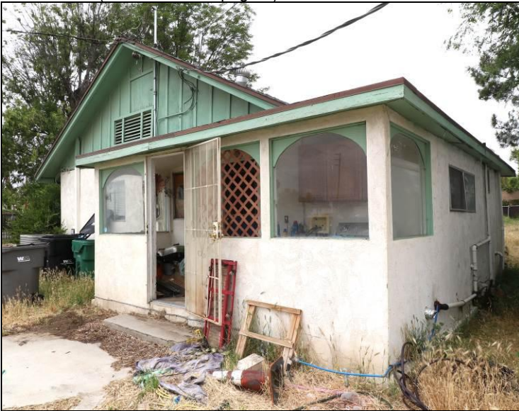
Addition on south and east elevations, view northwest (May 6, 2025).
