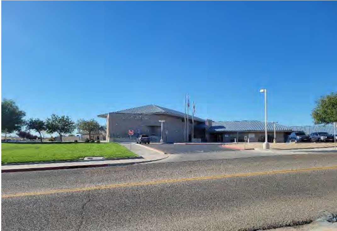
Photograph 1: Overview of the Challenger campus elevation, flat built environment. Photo facing south, taken October 10, 2024.
