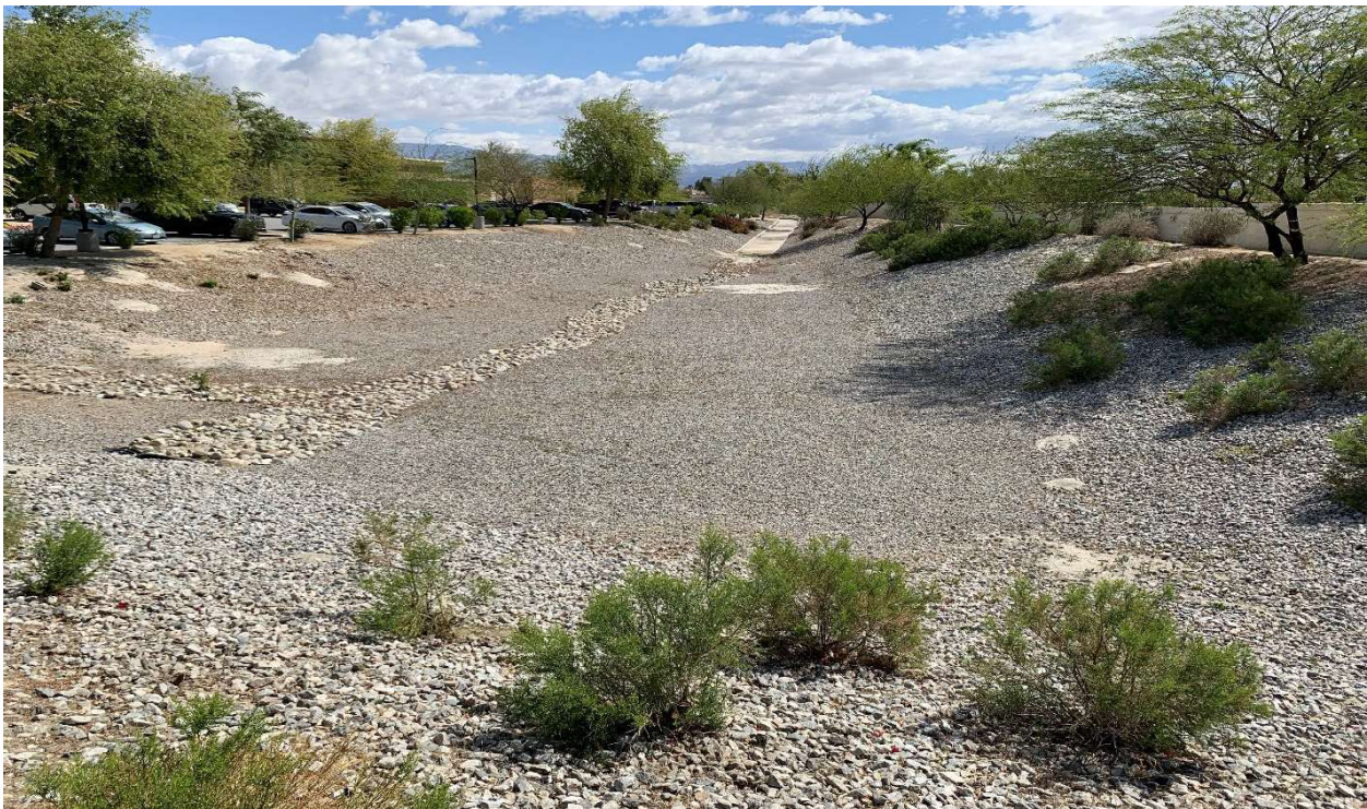
Photograph 10. East-facing view of area where flows from the underground storm drain outlet east of Da Vall Drive.
