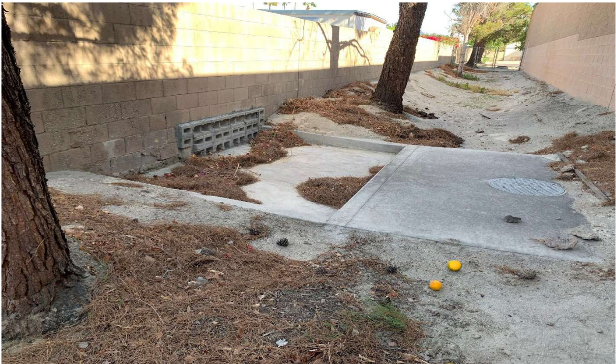
Photograph 4. View of concrete pad and flat, narrow culvert collecting road runoff from offsite, facing northwest.
