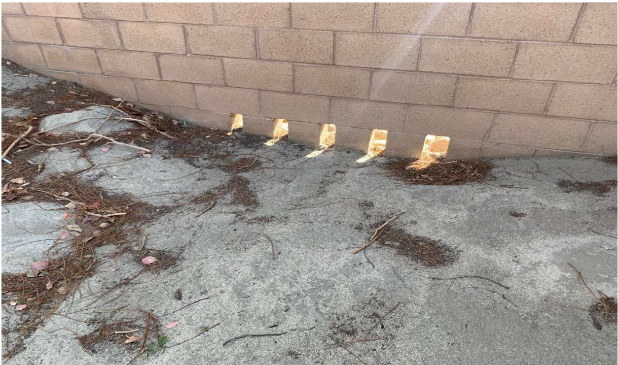
Photograph 8. View of east end of retention basin, where runoff exits through five gaps at the bottom of the brick wall.
