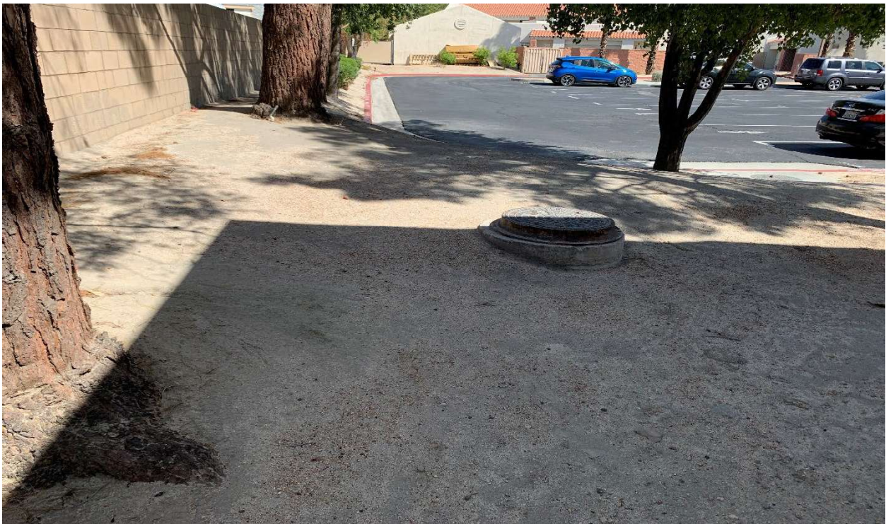
Photograph 2. A man-hole is shown in the landscaped area in between the shallow retention basins and the parking lot. No drainage feature or evidence of flows is present.
