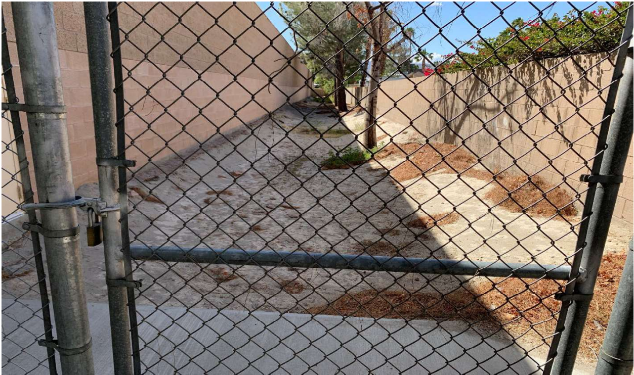
Photograph 3. South-facing view of chain-link fence and north end of the retention basin.
