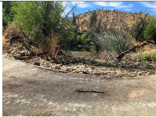
Adams Pond Spillway looking west at Pond (9/11/25).
