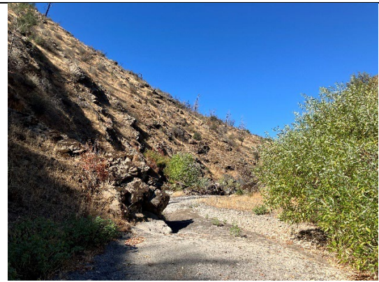
West end of the Project Limits, Stinking Creek, looking West (9/15/25).
