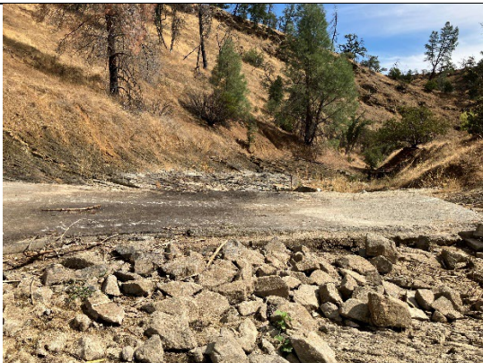
Adams Pond Spillway looking east, Stinking Creek downstream from Spillway (9/11/25).
