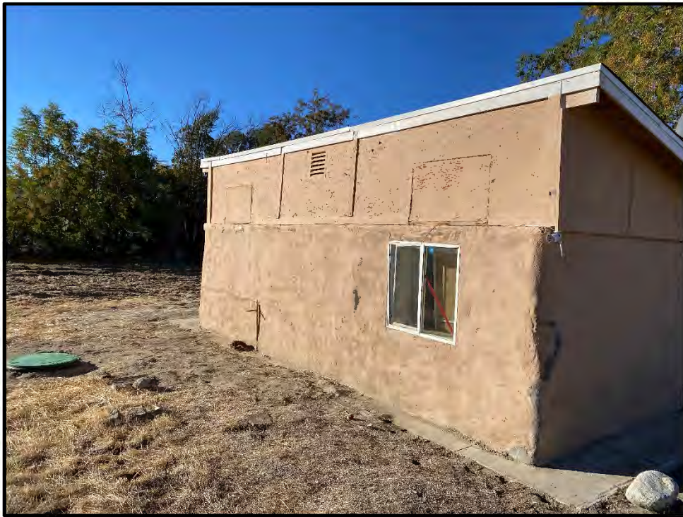
Plate 4.2-7: View of the east and north façades of the ancillary structure.
