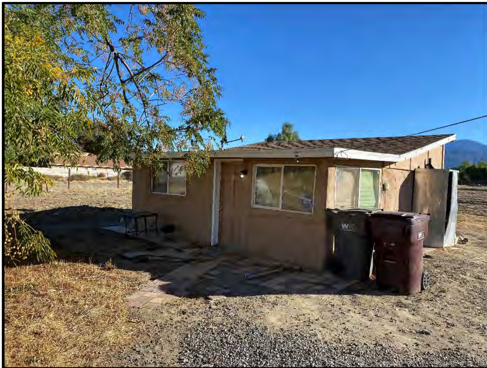
Plate 4.2–3: Western façade of the converted ancillary structure, facing northeast.
