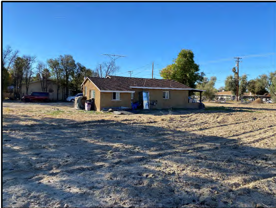
Plate 4.2–5: View of the north and east façades of the residence showing the addition and altered windows.
