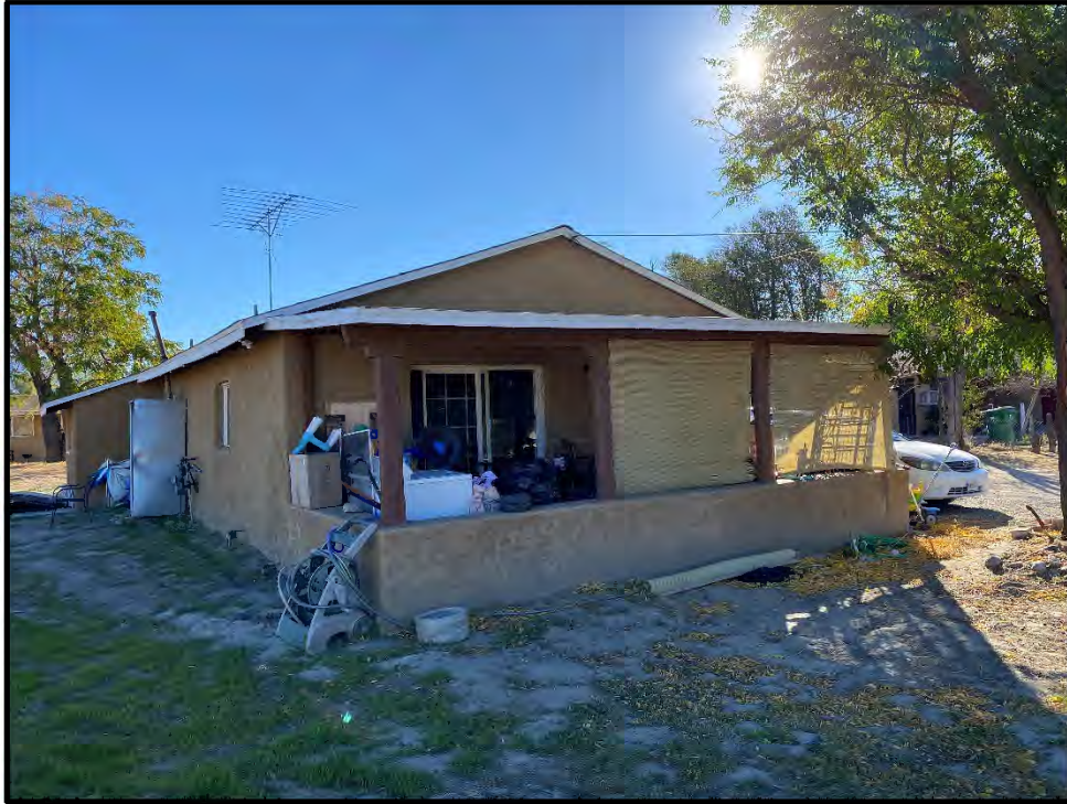
Plate 4.2–4: View of the west façade of the main residence.
